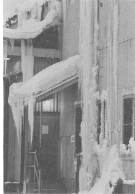
FIG. 27—Icings from roof meltwater.
