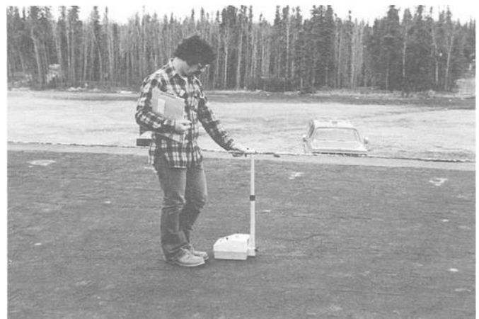
FIG. 34—Surveying a roof with a nuclear meter.
