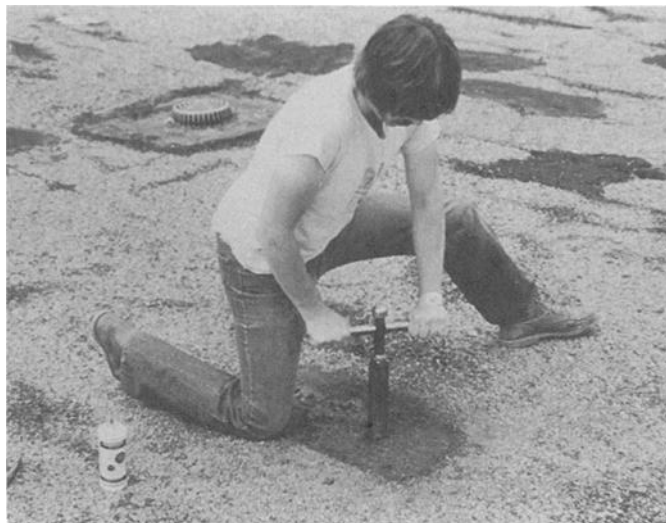
FIG. 40—Obtaining cores to verify a roof moisture survey.
