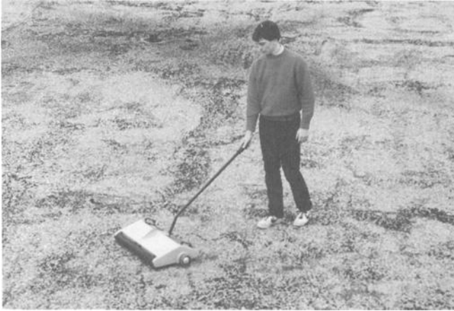
FIG. 35—Surveying a roof with a capacitance meter.
