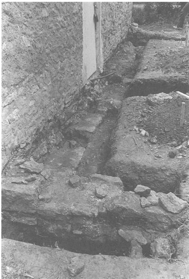
FIG. 5— In regrading to alleviate poor site drainage or excavating a foundation, archeological evidence may appear. Care should be taken to identify, record, and preserve important historic evidence. Photo: Milwaukee County Historical Society, NPS files.
