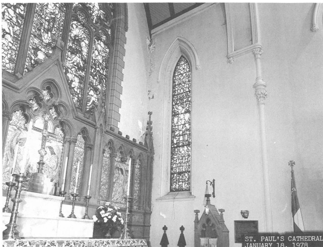
FIG. 16— Moisture damage on the interior may be a direct result of an exterior problem. In this case, the corner leak at the roof suggests that the internal downspout drain has become blocked. The use of a video camera, specially designed to look into drains, may help determine the condition of this internal drain. The exterior mortar of the masonry should also be inspected. Photo: NPS files.
