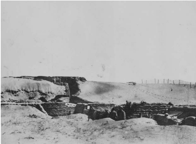
Figure 4.2 "British Trenches in the Sand Dunes on the Gaza Front." Note how the walls are shored up or "revetted" by sandbags to hold the sand in place. Official British pictures of the First World War, 1914–18 (Crown Copyright), US Library of Congress, Lot 7882-1, #85
