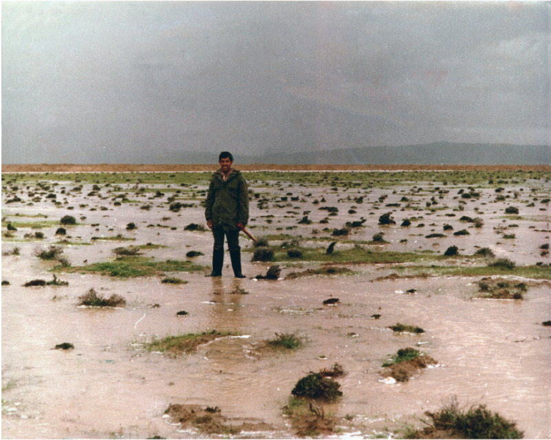
Fig. 1 The faint, straight line in the upper part of the picture is the conveyor-spreader channel that flows from right to left. In this event, which occurred on 6 March 1983, 5 \text{ m}^3\text{s}^{-1} of floodwater was spread along 1,000m of this 1,342m canal. The mean depth over the sedimentation basin was 5 cm, and the velocity was 20 \text{ cm}^{-1} .
