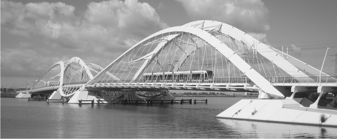
Figure 2-1. Enneüs Heerma Bridge (with tram) between Amsterdam and Island of IJburg, the Netherlands. (Courtesy of S. Sepp.)
