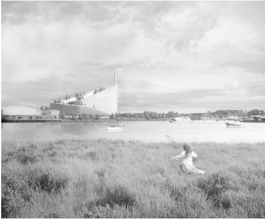
Figure 5-5. Rendering of the Amager Bakke Combined Heat and Power Waste-to-Energy Plant, with ski slope, Copenhagen, Denmark. (Courtesy Bjarke Ingels Group.)
