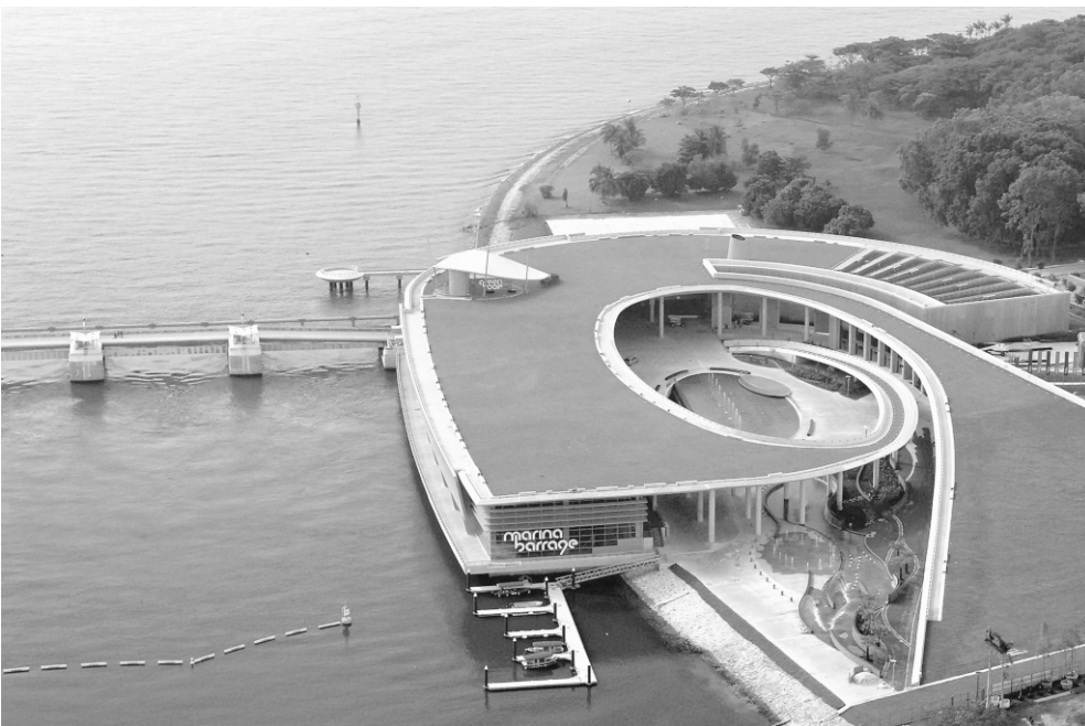
Figure 7-3. Aerial view of Marina Barrage and Visitor Centre, Singapore. (Courtesy of CDM Smith.)
