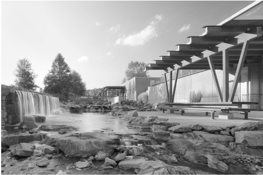
Figure 5-6. Willamette River Water Treatment Plant from downstream, Wilsonville, Oregon (© Nic Lehoux).
