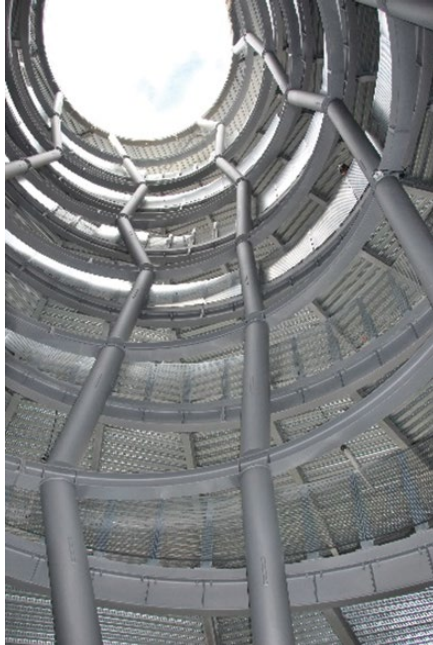
Figure 1 Inside view of the access route in the carpark. © ConstruirAcier.
