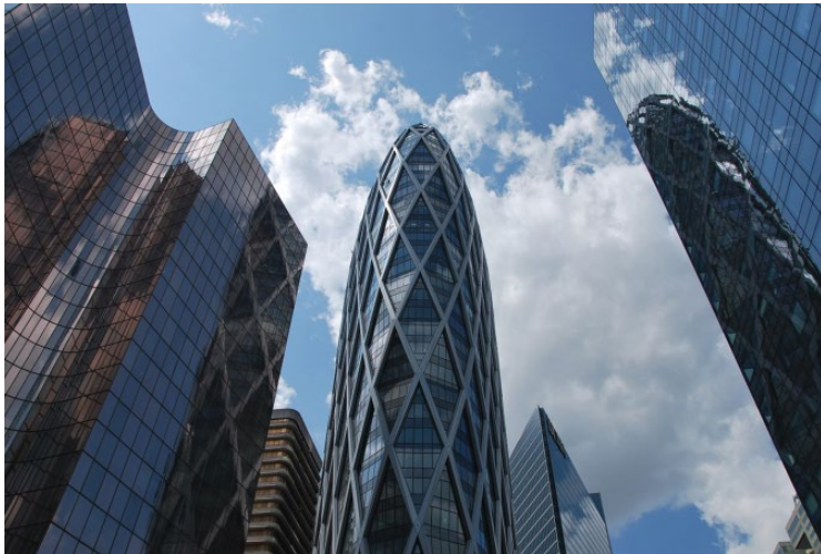
Figure 3 External diagrid structure with its diamond-shaped windows creates a unique lighting effect. © ConstruirAcier.
