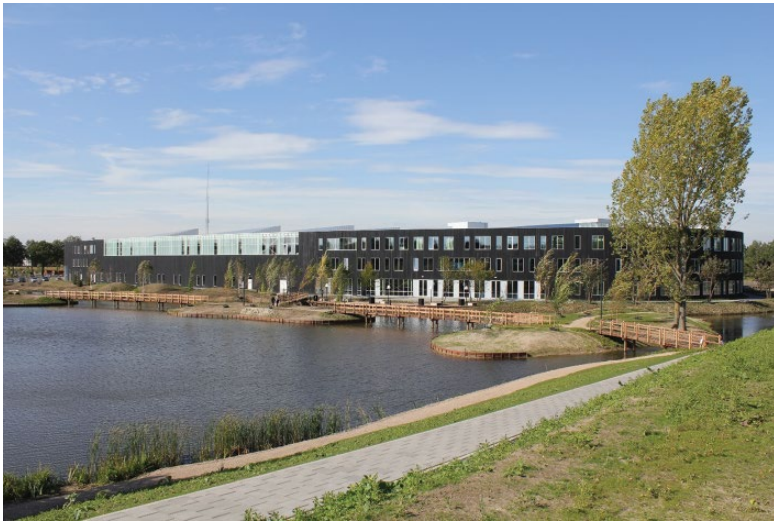
Figure 1 Venco Campus Eersel. © Slimline Buildings.
