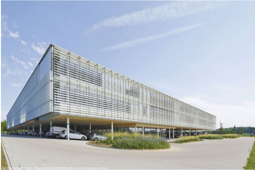
Figure 3 Slipped under the offices following the natural gentle slope (1.5%–2.5%), the parking area is discreetly positioned under the building, preserving the surrounding landscape. © Jean-Michel BYL.
