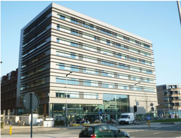
Figure 1 Amstelcampus Boerhaave complex, Amsterdam. © Slimline Buildings.
