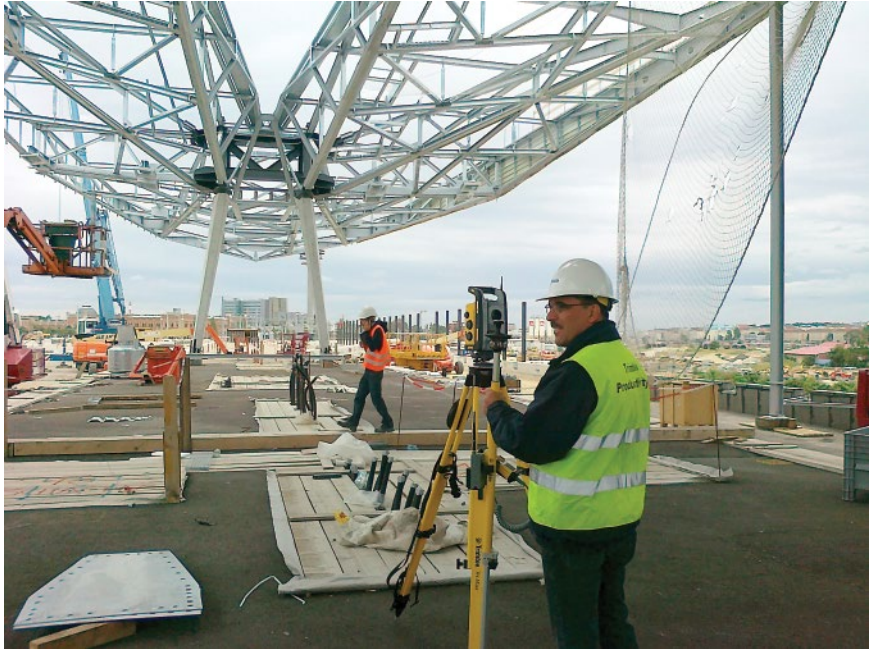
Figure 3.10 With the help of the Trimble total station and the data from the BIM model, the roof elements were precisely positioned. © Trimble.
