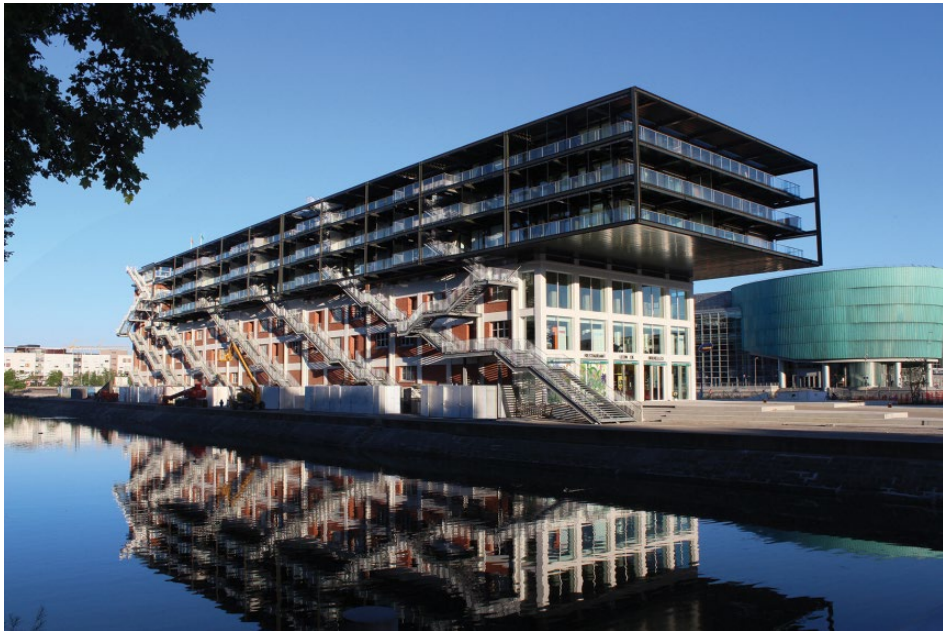
Figure 1 On the northern facade, fire escapes are externalized, connecting the different uses with some structural acrobatics. © Heintz-Kehr Architectes.
