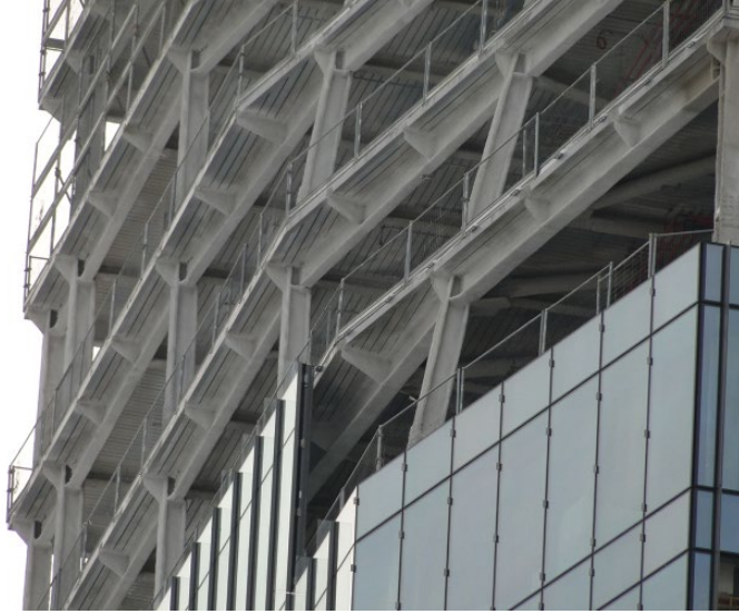
Figure 2 Steel structure with inclined columns. © bauforumstahl.
