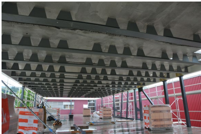
Figure 3 TOPfloor INTEGRAL elements with large openings for easily accessible installation. © H. Wetter AG.
