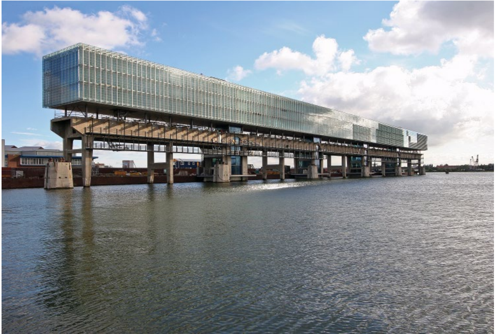
Figure 3.16 Kraanspoor project in Amsterdam harbour. Three storeys of lightweight steel structure on top of an existing concrete frame. © Initiative and design: Trude Hooykaas, architect: OTH architects, photographer: Rob Hoekstra.
