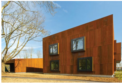
Figure 1 View of the south façade. © Gilles Martin.
