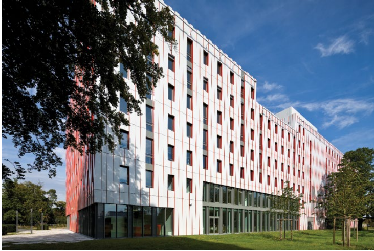
Figure 2 Aluminium cassette facade – the facade changes colour from grey to red depending on the perspective. © Goldbeck.
