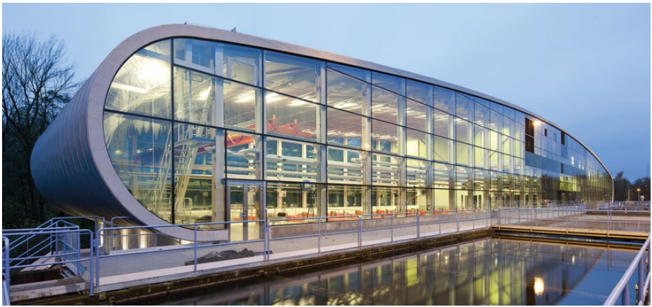
Figure 1 Rya Wastewater Treatment Plant. © Kasper Dudzik.
