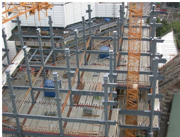
Figure 2 Construction site – the steel structure is visible. © Slimline Buildings.
