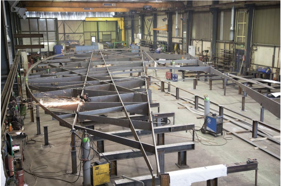
Figure 3.13 The roof was prefabricated in the workshop, then divided into seven transportable segments and assembled on the ground immediately next to the final location. © Ingo Schrader Architekt BDA.
