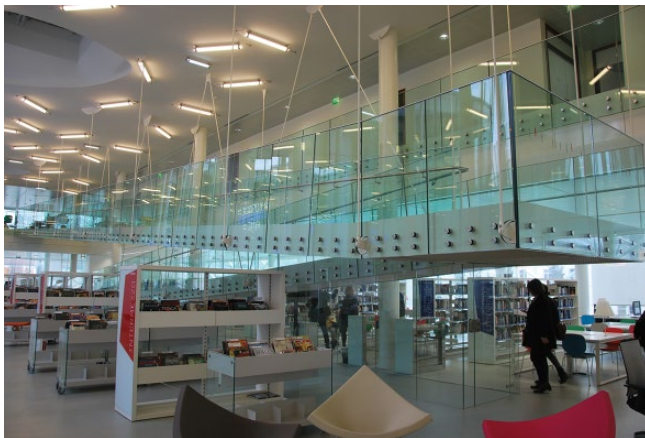
Figure 2 Suspended footbridge inside the library building. © ConstruirAcier.
