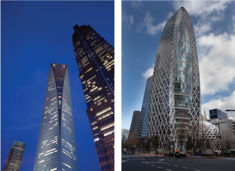
Figure 4.51 Intumescent coatings are used, for example, in the World Financial Center and Jin Mao Tower in Shanghai (left) and in the Mode Gakuen Cocoon Tower in Tokyo (right). © AkzoNobel.
