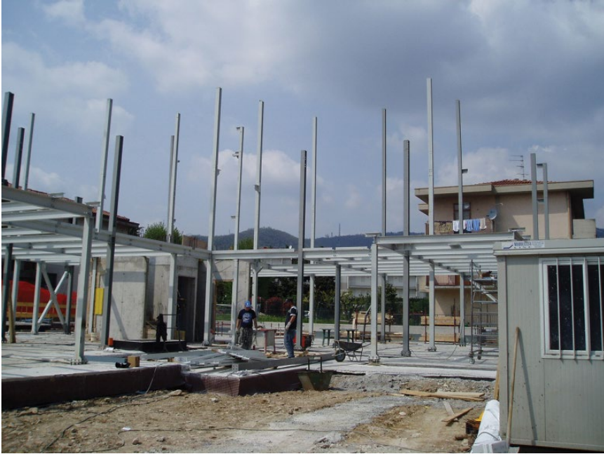
Figure 2 Construction site – the steel structure is still visible. © Atelier2 – Gallotti e Imperadori Associati.
