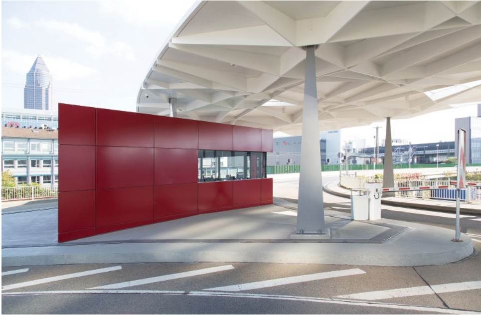
Figure 3.14 Oval roof of the north entrance of the Frankfurt trade fair grounds, Architecture: Ingo Schrader Architekt BDA, Structural Design, Physics and Sustainability: Bollinger + Grohmann. © Ingo Schrader Architekt BDA.
