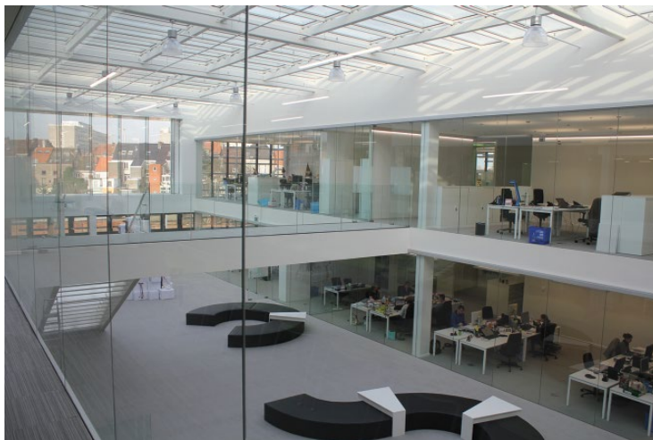
Figure 2 16.2 m column-free spans. © Slimline Buildings.
