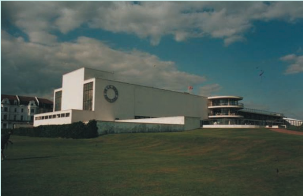
Figure 10.2 The de la Warr Pavilion at Bexhill-on-Sea, East Sussex – designed by Mendelssohn and Chermayeff in the 1930s and now considered the finest example of modernist architecture in Britain – draws tourists to an otherwise declining seaside resort. (Photo by Chris Holloway.)
