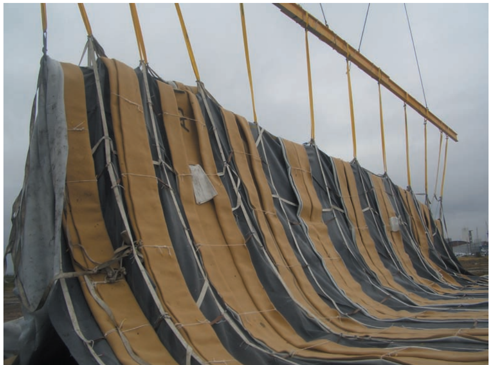
Figure CS9.3 The artificial reef is hoisted prior to its positioning offshore. (Courtesy of Bournemouth Tourism.)
