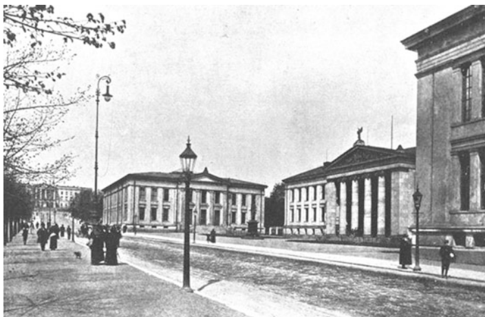
Fig. 1.2 The Royal Frederiks University of Kristiania. The main street of Kristiania/Oslo, Karl Johan started at the Royal Castle and passed in front of the University. This picture was taken about 1900. The three main University buildings open officially in 1851. The middle building with a column façade, is called the Domus Media
