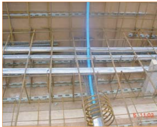
Figure 7.39 Typical dead end anchorage showing the grout tube and bursting helix (courtesy of Sir Robert McAlpine Ltd)
