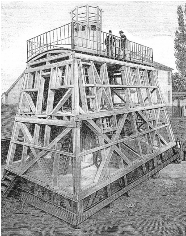
Fig. 12.6 The Mont Blanc Observatory assembled at Meudon before transport. La Science Illustrée, 1893. © Paris Observatory Library
