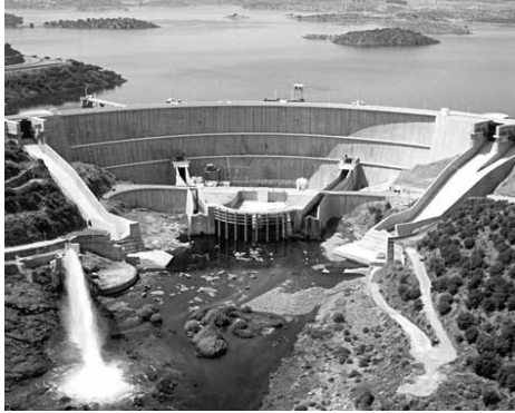
Figure 1: Alqueva dam: view from downstream to upstream.
