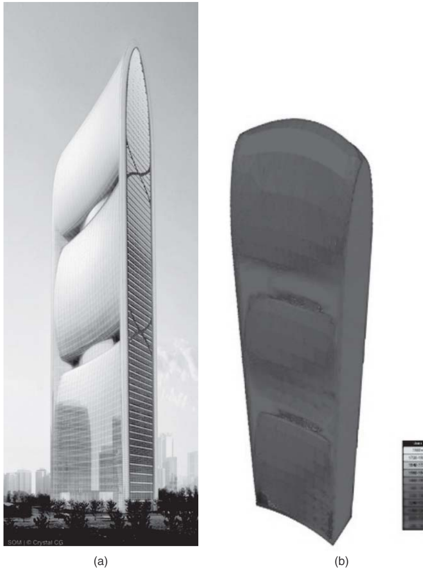
Figure 1.9 Building information modeling uses computer technology to create a virtual model of a building as an integrated part of the design process. (a) The design of the Pearl River Tower designed by Skidmore, Owings & Merrill, LLP, for construction in Guangzhou, China, includes integrated wind turbines and photovoltaic panels to offset its energy use. (b) Ecotect model showing the amount of solar radiation on the tower's various surfaces.
