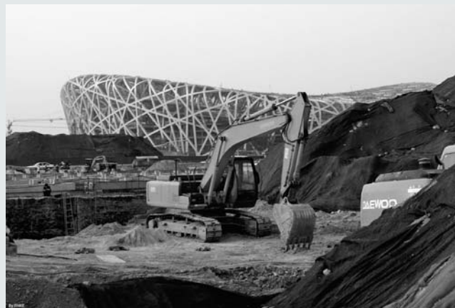
Figure S2.6 Construction of Beijing Olympic Stadium.
