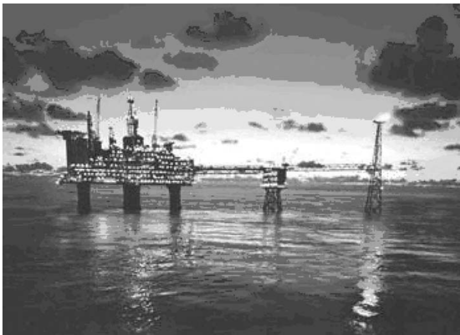
Figure 7.9 Carbon dioxide that is produced at the Sleipner natural gas complex off the coast of Norway is removed and pumped into the Utsira Formation, a highly permeable sandstone. In this case, the sequestration cost is less than the Norwegian carbon emission tax. Courtesy of Øyvind Hagen, Statoil.
