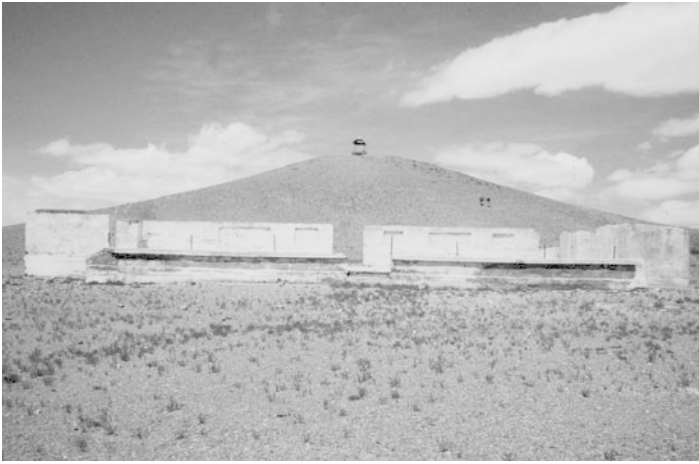
Figure 4.1 Dismantled community center near Ölziit Sum, Dundgov' Aimag, 1996. Many such buildings in rural Mongolia were stripped for materials by locals once Soviet subsidies for sum centers disappeared after 1990.
