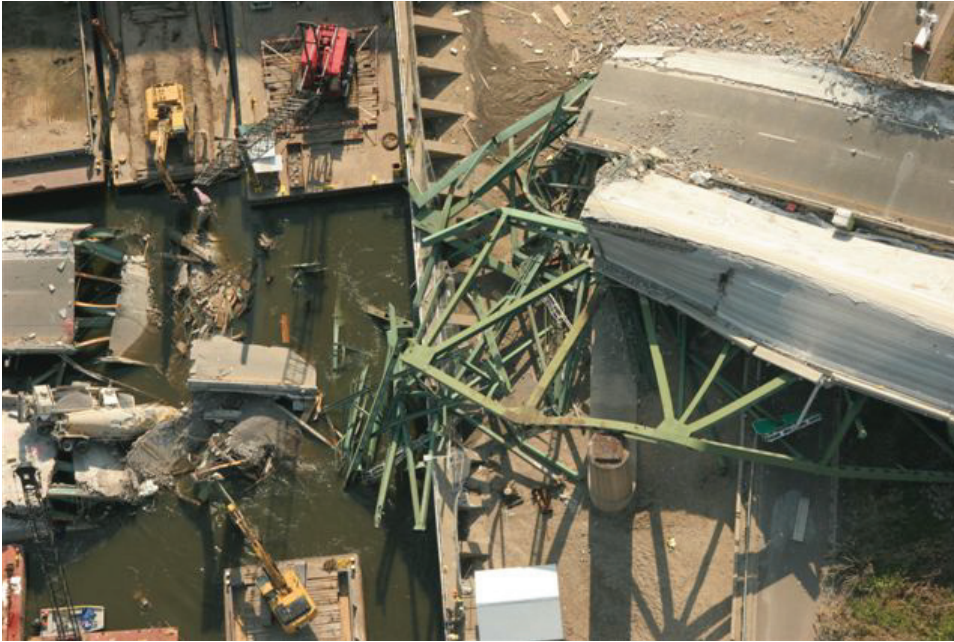
FIGURE 1.1 The scene of the collapse of the I-35W bridge in Minneapolis, Minnesota, in 2007. SOURCE: Minnesota Department of Transportation. Available at http://www.dot.state.mn.us/i35wbridge/photos/aerial/aug-16/index.htm .
