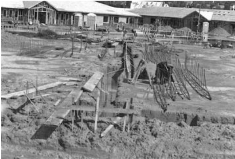
FIGURE 16.4 Footing excavations. Note the flooded condition of the footing trenches.
