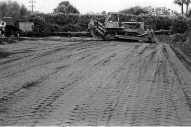
FIGURE 15.3 A lift of fill has been placed and compacted into a dense state.
