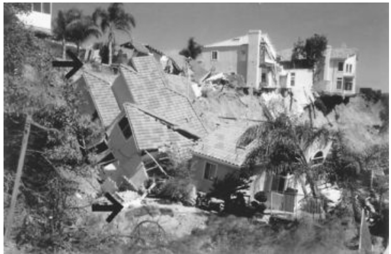
FIGURE 10.34 Laguna Niguel landslide: head of the landslide. ( Note: The vertical distance between the two arrows is the distance that the landslide dropped downward.)
