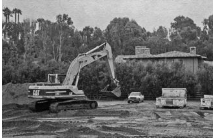
FIGURE 15.12 The excavator is ideally suited to excavating narrow trenches for the construction of utilities such as storm drain lines and sewer lines.
