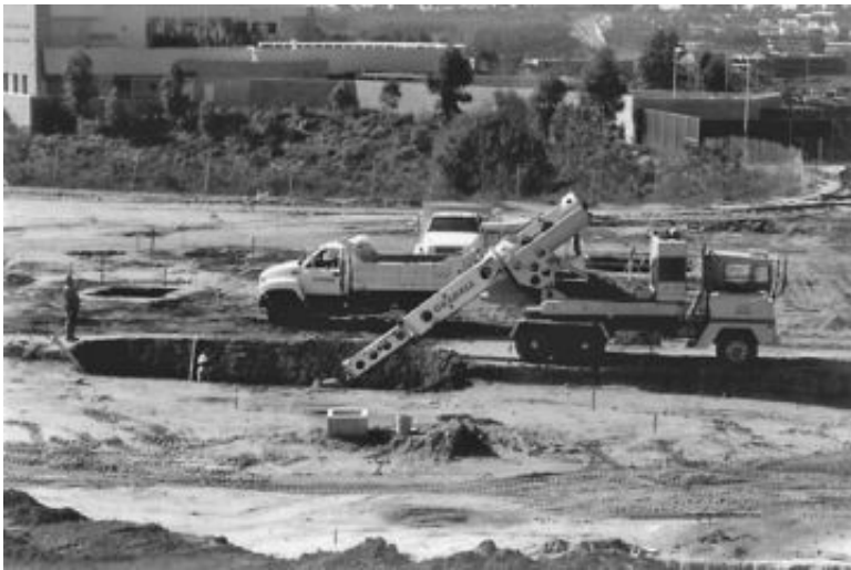
FIGURE 16.2 Excavation of footings.
