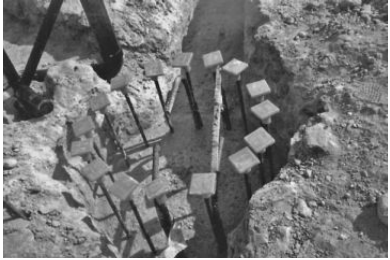
FIGURE 16.13 The pier hole has been filled with concrete. The steel reinforcement from the pier will be attached to the steel reinforcement in the grade beam.
