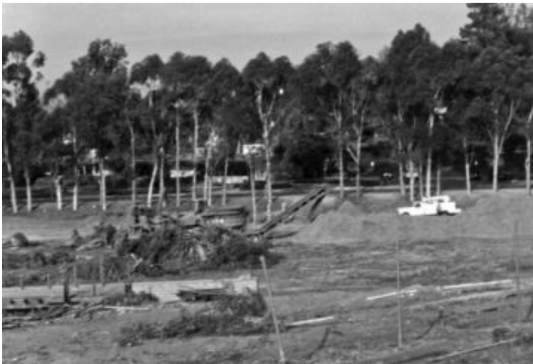
FIGURE 15.2 A large mechanical grinder has been brought to the site and the trees and brush are being ground-up into wood chips. The wood-chips will be removed from the site and then recycled.
