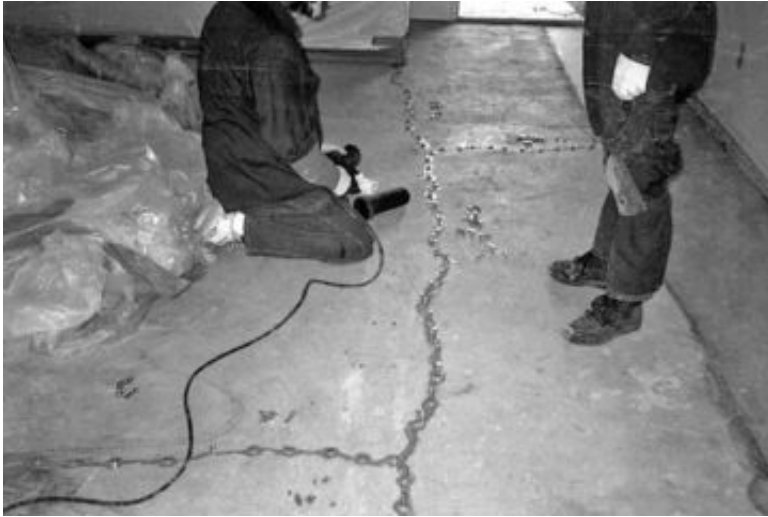
FIGURE 16.47 Pressure injection of epoxy into concrete slab cracks.
