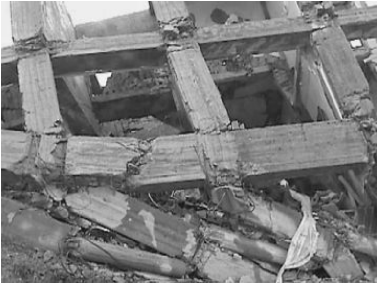
FIGURE 14.5 Building collapse caused by a soft story at the first-floor level. The damage occurred during the Kocaeli earthquake in Turkey on August 17, 1999. (Photograph by Mehmet Celebi, USGS.)
