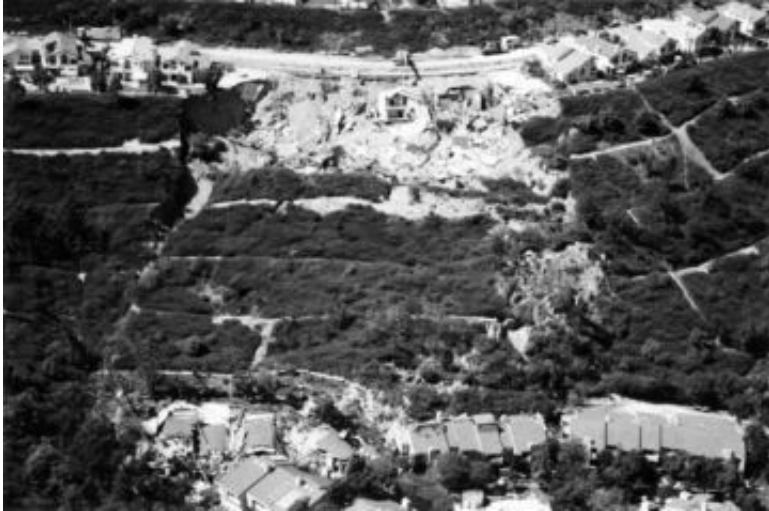
FIGURE 10.27 Overview of the Laguna Niguel landslide.
