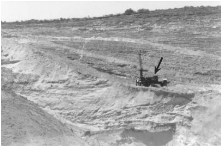
FIGURE 2.28 Access road constructed for subsurface investigation at an open-pit mine (arrow points to bucket auger drill rig).
