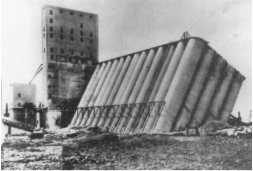
FIGURE 6.4 Transcona grain elevator failure.
