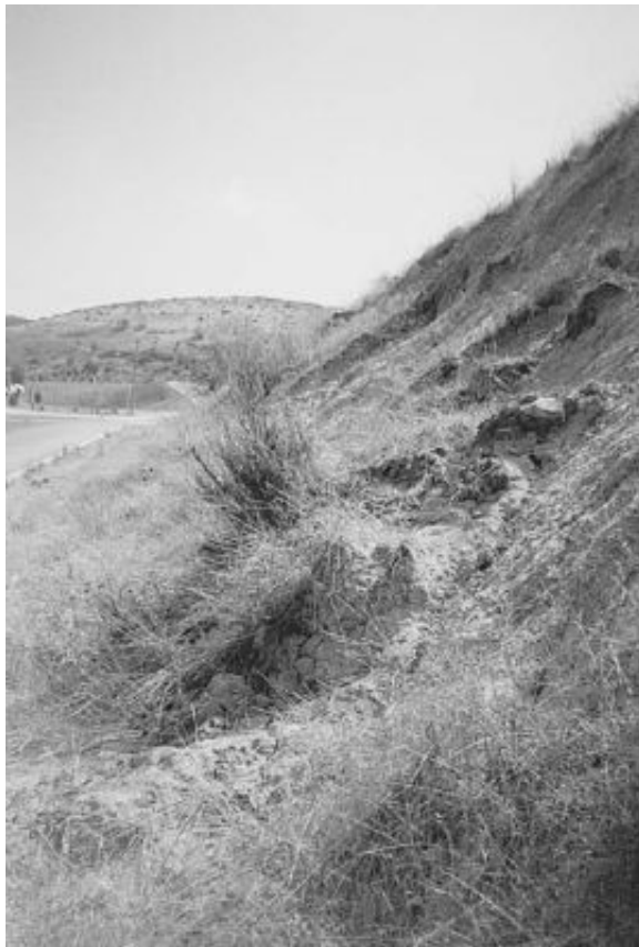
FIGURE 10.12 Surficial failure, cut slope for road.
