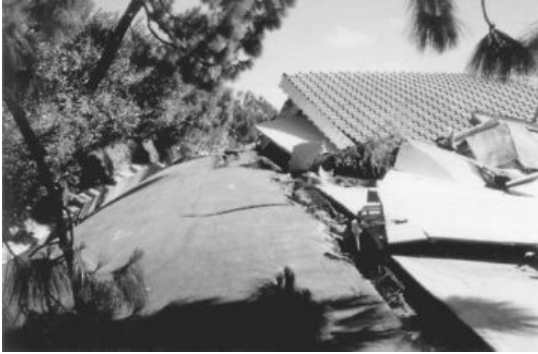
FIGURE 10.31 Laguna Niguel landslide: view of the toe of the landslide where the road has been uplifted 20 ft.
