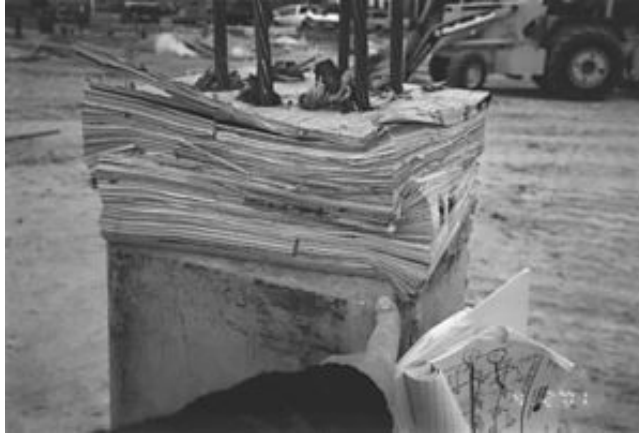
FIGURE 6.11 Close-up view of Fig. 6.10. The wood cushion blocks have been crushed together during the pile driving operation.
