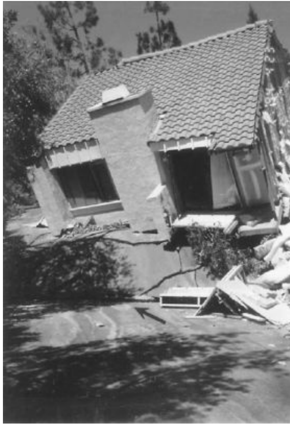
FIGURE 10.30 Laguna Niguel landslide: view of the toe of the landslide (note that the arrow indicates the original level of this area, but the landslide uplifted both a portion of the road and the condominium).
