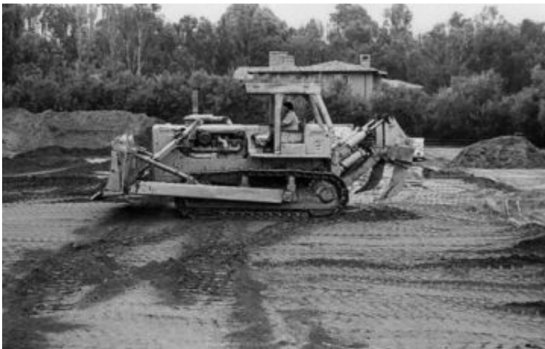
FIGURE 15.9 The bulldozer is in the process of spreading out a layer of fill for compaction.
