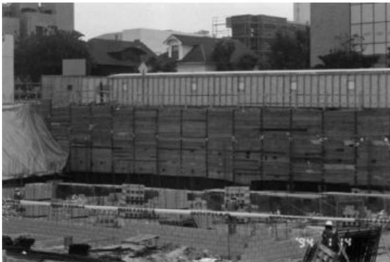
FIGURE 11.19 Temporary steel I-beam and wood lagging retaining wall having tieback anchors. The temporary retaining wall is being used to support the excavation during the construction of the foundation.
