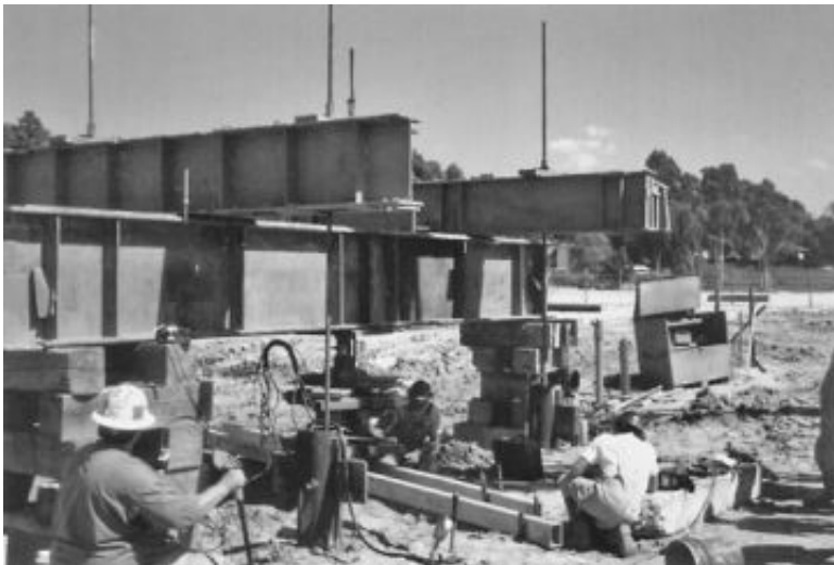
FIGURE 16.34 Pile load tests. The reaction frame has been set up and the hydraulic jack and load cell are in place.
