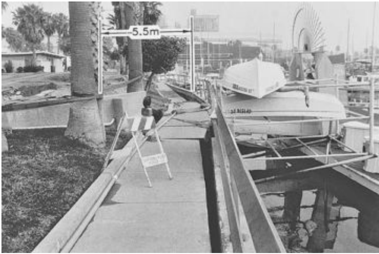
FIGURE 13.19 Damage to a marine facility caused by the California Northridge earthquake on January 17, 1994. (From Kerwin and Stone, 1997; reprinted with permission from the American Society of Civil Engineers.)
