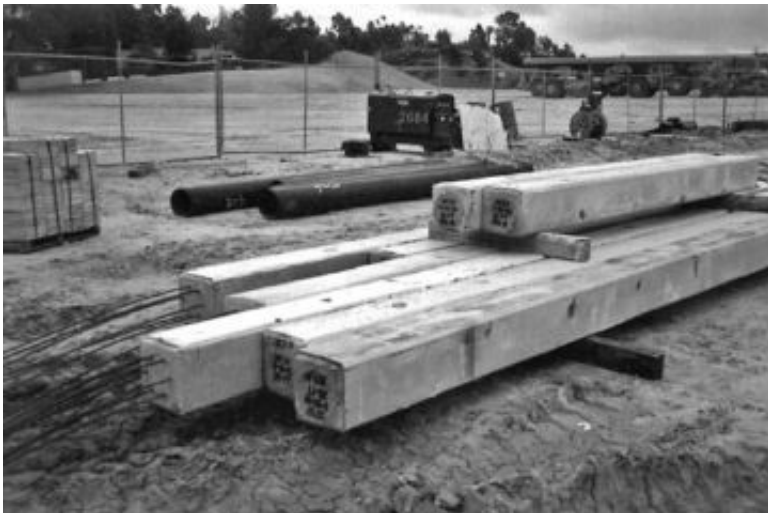
FIGURE 16.21 Prestressed concrete piles stockpiled at the job site.
