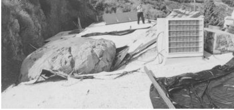
FIGURE 10.4 Rockfall in Santiago Peak volcanics.
