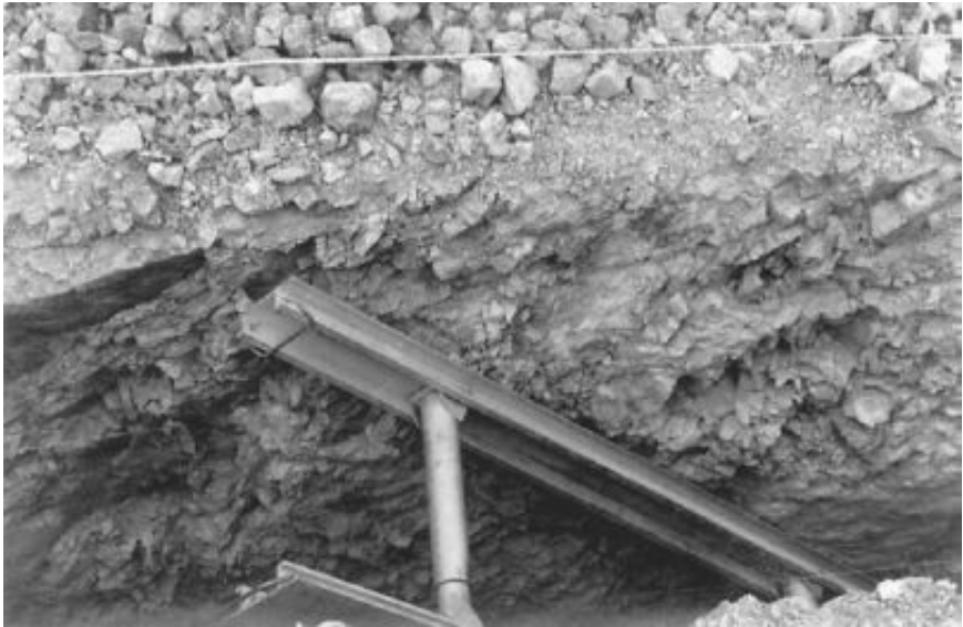
FIGURE 2.31 Close-up view of trench excavation.
