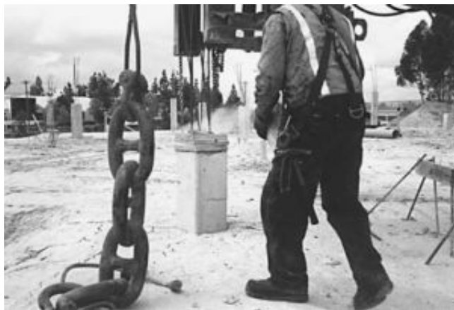
FIGURE 6.10 The prestressed concrete pile at the center of the photograph is the same pile as shown in Fig. 6.9 and has just been driven into place. Note that the cushion blocks of wood have been compressed during the pile driving. The steam emanating from the wood is due to heat generated during the impact with the hammer.
