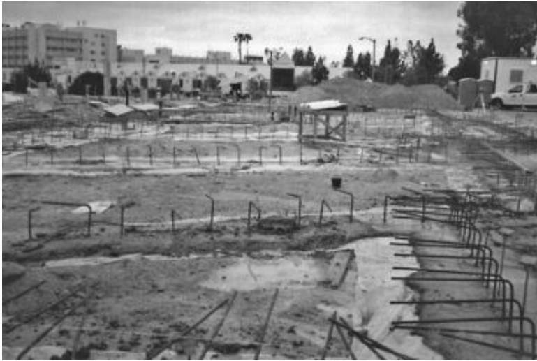
FIGURE 16.17 The concrete for the grade beams has been placed. The steel reinforcement from the grade beams will be attached to the steel reinforcement in the floor slab.
