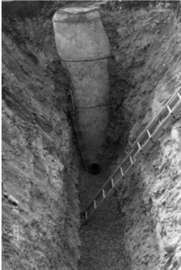
FIGURE 15.7 Utility trench excavation for a storm-drain line.
