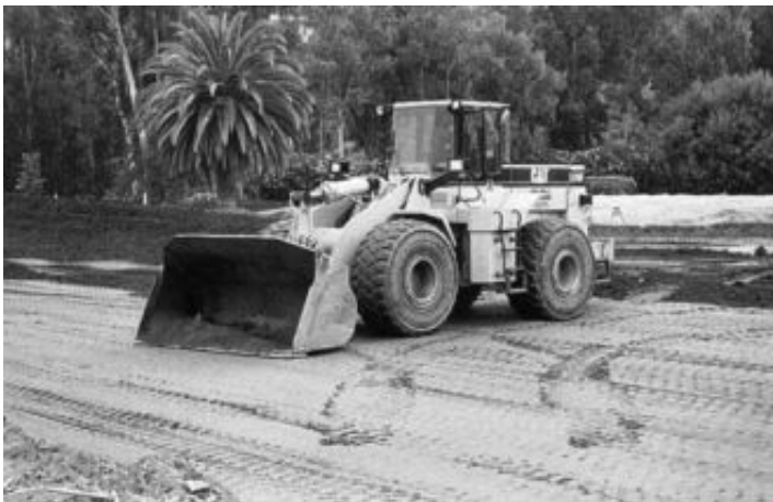
FIGURE 15.11 The loader can be used to move soil about the job site and compact the soil as structural fill.
