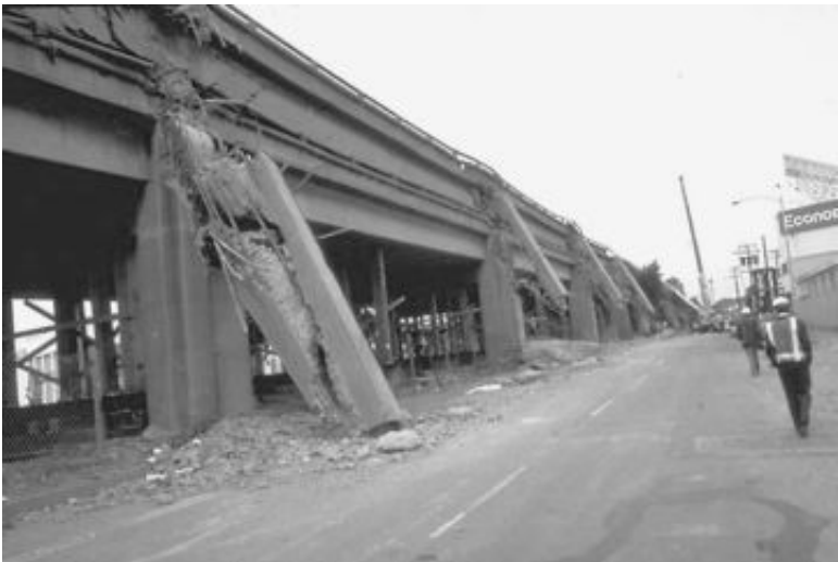
FIGURE 13.13 Close-up view of the collapse of the Cypress Street Viaduct caused by the Loma Prieta earthquake in California on October 17, 1989. (From USGS.)
