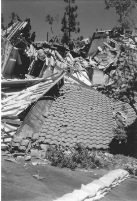
FIGURE 10.33 Laguna Niguel landslide: view of damage at the toe of the landslide. The landslide has crushed the buildings located in this area.
