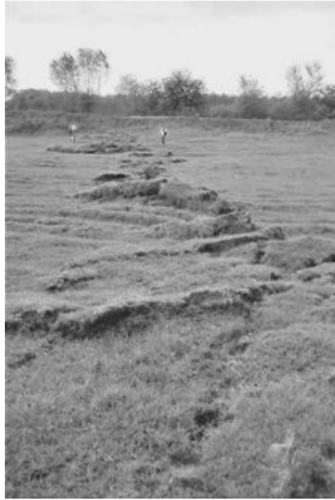
FIGURE 13.4 Surface fault rupture associated with the Kocaeli (Turkey) earthquake on August 17, 1999 (Photograph by Tom Fumal, USGS.)
