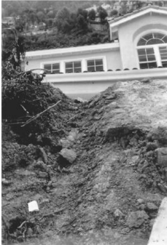
FIGURE 10.39 Laguna Niguel landslide: head of the landslide showing a house that has been pulled downslope.
