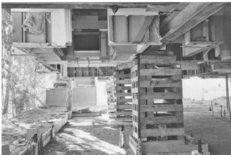
FIGURE 16.40 Construction of the mat foundation.
