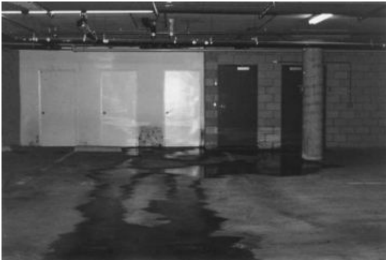
FIGURE 11.22 Overview of the same area shown in Fig. 11.21.
