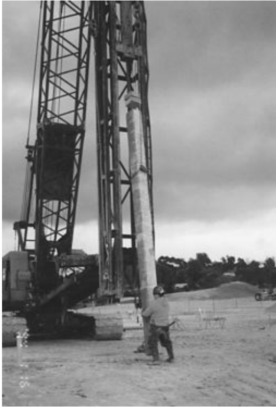
FIGURE 6.9 A prestressed concrete pile is being hoisted into place for driving. Wood blocks have been placed at the top of the pile to cushion the impact of the drive hammer and prevent damage to the top of the pile.
