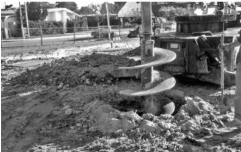
FIGURE 16.10 Close-up of auger being pushed into the soil.
