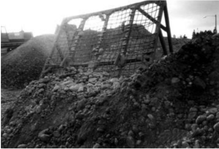
FIGURE 15.5 A screen has been set up in order to remove large-size rock fragments from the soil.
