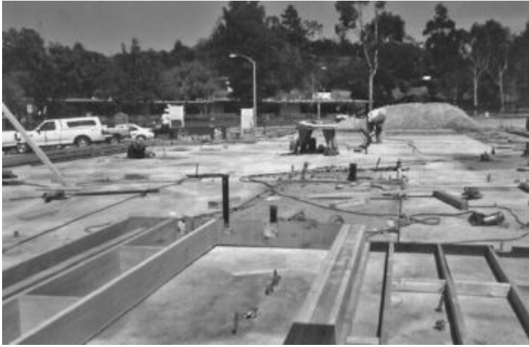
FIGURE 16.19 Concrete for the floor slab has been placed.
