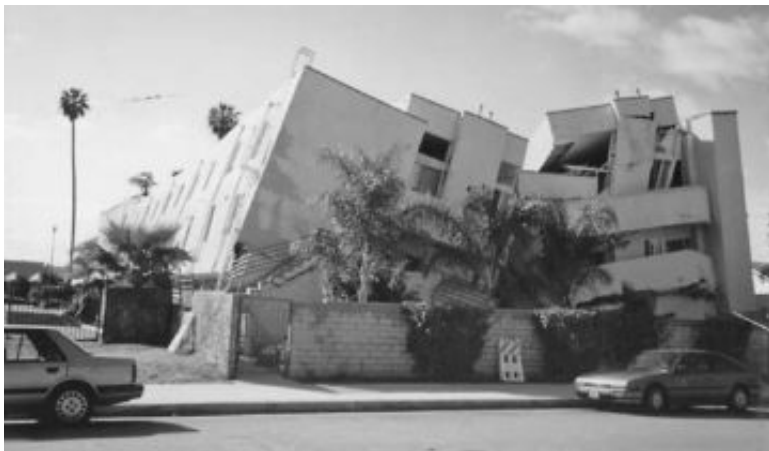
FIGURE 14.2 Building collapse caused by a soft story due to the parking garage on the first floor. The building collapse occurred during the Northridge earthquake in California on January 17, 1994.
