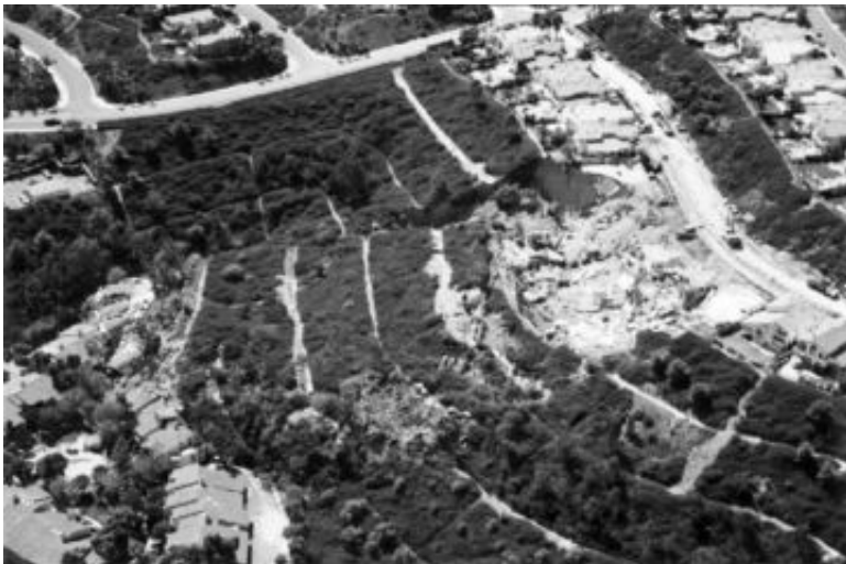
FIGURE 10.28 Overview of the Laguna Niguel landslide.
