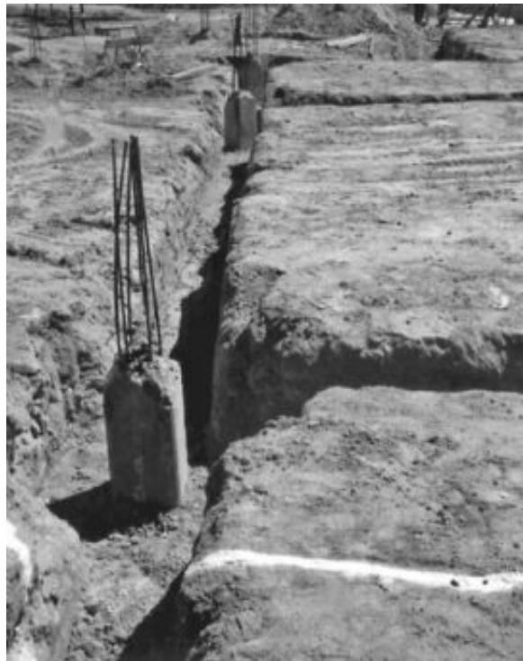
FIGURE 16.26 Prestressed concrete piles have been installed and the excavations for the pile caps and grade beams are complete. The strands at the top of the pile will be connected to the steel reinforcement in the pile cap and grade beam.
