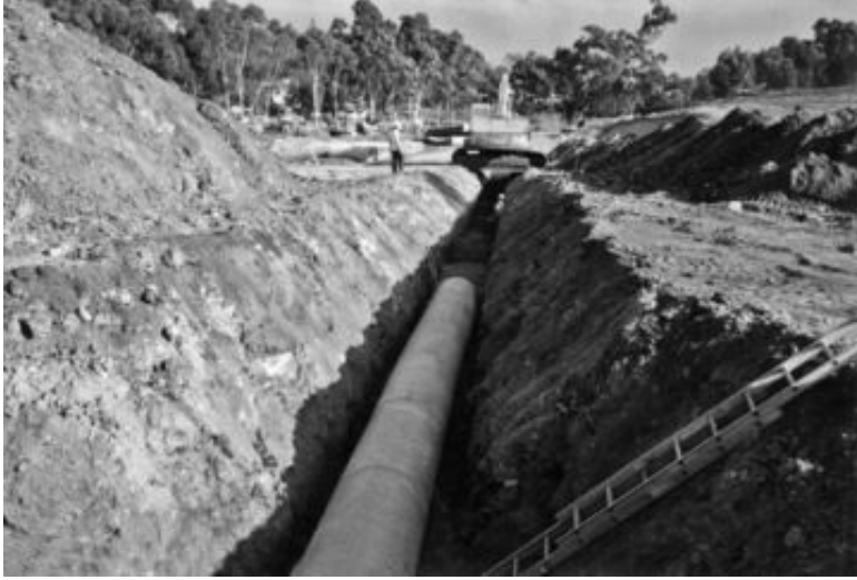
FIGURE 15.8 Another example of a utility trench excavation for a storm-drain line.
