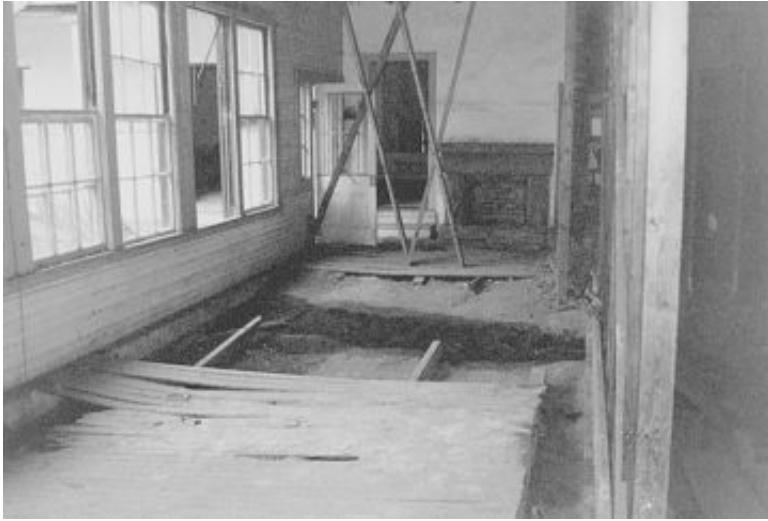
FIGURE 12.9 Drainage beneath parlor.
