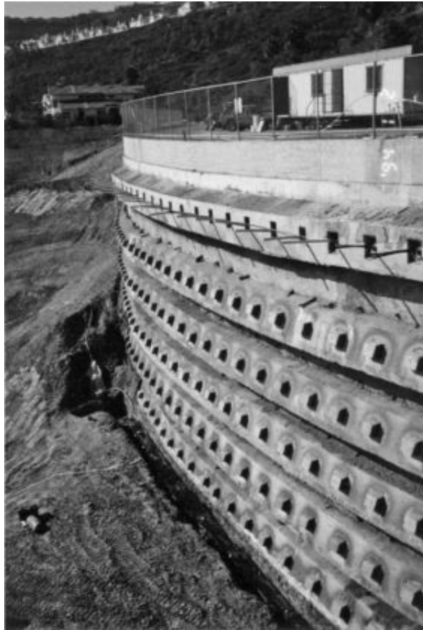
FIGURE 10.42 Retaining wall constructed at the head of the Laguna Niguel landslide.
