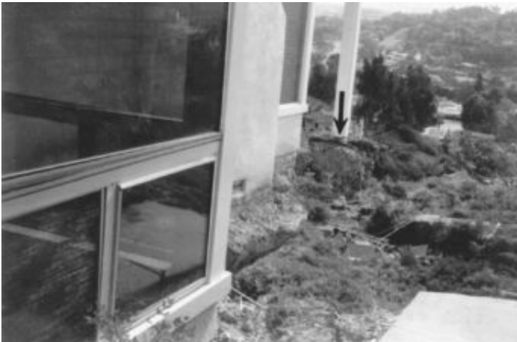
FIGURE 10.36 Laguna Niguel landslide: head of the landslide showing another house with a portion suspended in mid-air. (Note: The arrow points to a column and footing that are suspended in midair.)
