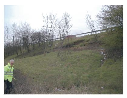
*Figure 3-9.* Shallow rotational slide affected by changes in pore pressures on an embankment of the M25, near London, UK (Photo: J.E. Norris).
