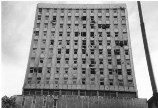
FIGURE A-2. Sarajevo State Hospital.
