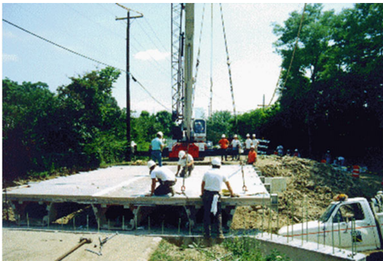
Fig. 16.3 All three sections of the Tech 21 Bridge installed
