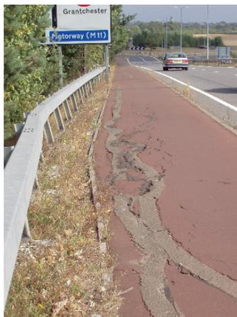
*Figure 5-6.* Embankment shrinkage due to the presence of high water demand trees (mainly oaks) on the overbridge at Junction 12, M11, U.K. (Photo: Courtesy of C. Bull, URS Corporation Ltd, Bedford, U.K.).
