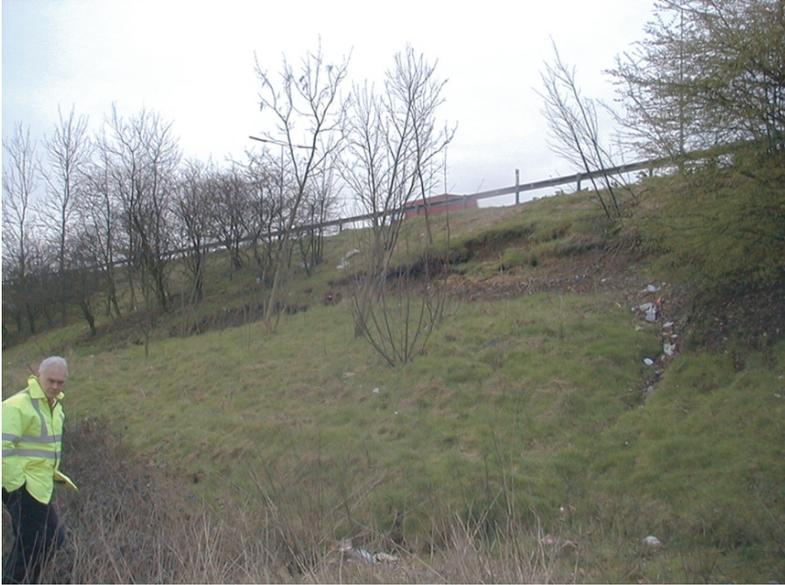
Figure 3-9. Shallow rotational slide affected by changes in pore pressures on an embankment of the M25, near London, UK (Photo: J.E. Norris).
