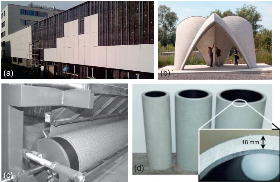
Figure 2.1 Examples of TRC use in prefabrication: (a) façade panels; (b) light shell elements (Ehlig et al., 2012); (c) application of textile reinforced concrete on a thin polymeric pipe (Lieboldt et al., 2008); and (d) cross-section of the hybrid pipe wall (six layers of reinforcement) (Lieboldt et al., 2008).
