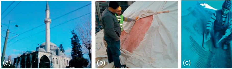
Figure 17.19 Strengthening the masonry dome of Molla Çelebi Mosque: (a) the mosque; (b) application of “Horasan” mortar on the outside of the dome; and (c) application of the textile basalt grid over a layer of cementitious mortar. Kind permission of Fyfe Europe SA.
