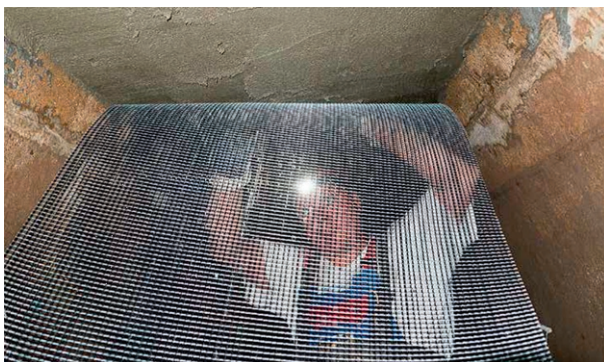
Figure 12.14 Sewer restoration with TRC in Dresden (Walther and Curbach, 2015).
