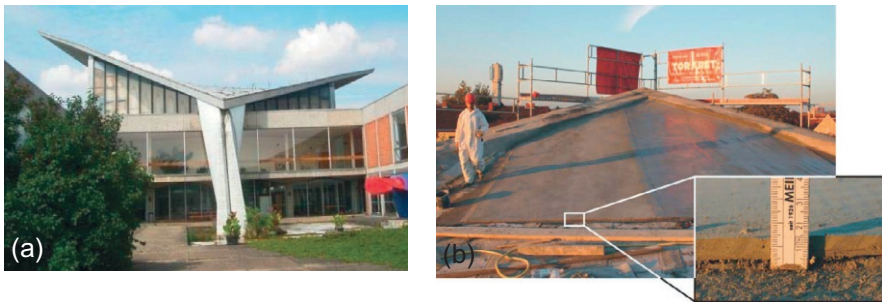
Figure 6.2 (a) Damaged steel-reinforced concrete hyper-shell at the FH Schweinfurt (Germany) and (b) strengthening with TRC (Weiland et al., 2008).
