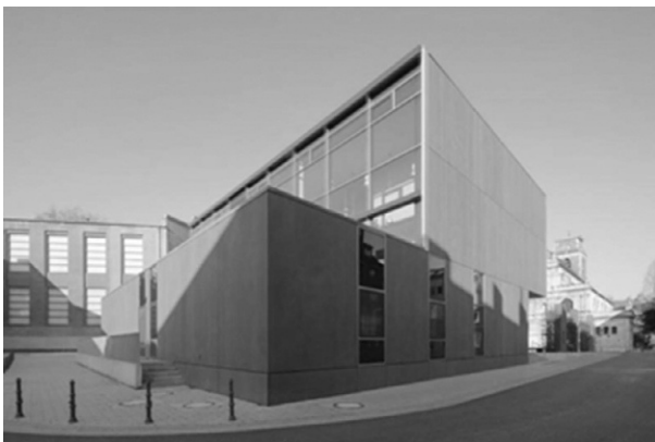
Figure 10.1 Large façade panels covering part of the lateral envelope of the St. Leonhard school building.
