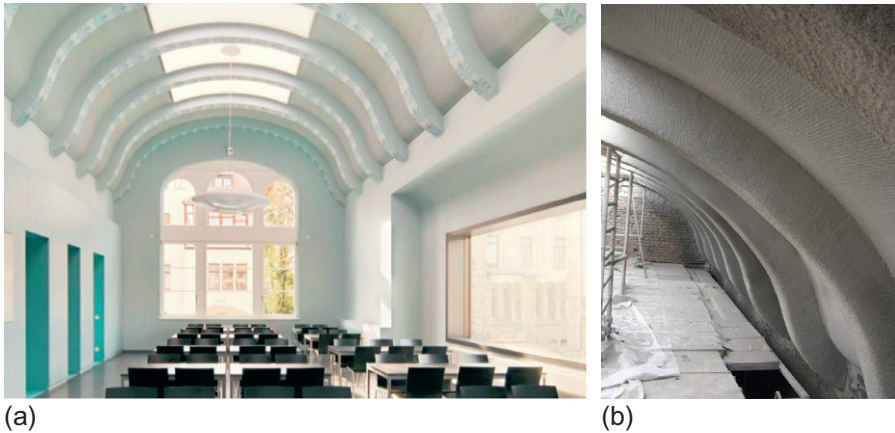
Figure 12.10 The tax office in Zwickau, Germany. (a) The completed reinforced barrel vaulting (Erhard et al., 2015) and (b) the sprayed TRC layer (TORKRET GmbH).
