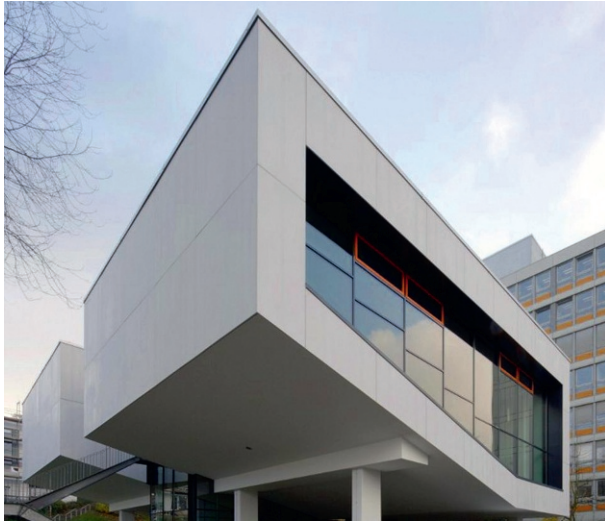
Figure 12.4 View of the auditorium of the Civil Engineering Faculty, RWTH Aachen University (Grebe, 2011).
