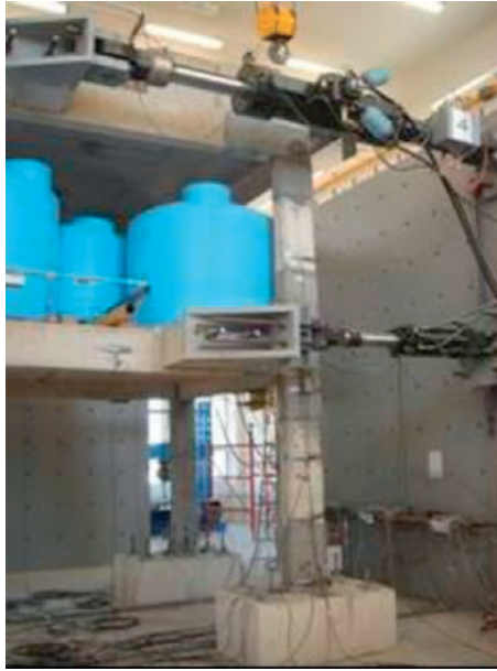
Figure 13.17 Pseudodynamic testing of two-story RC building retrofitted at column ends with TRM jacketing.
