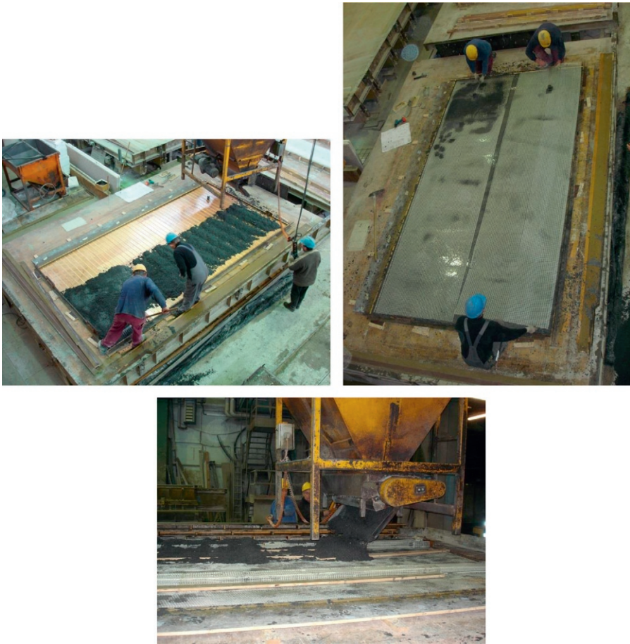
Figure 3.7 Manufacturing a façade element.
