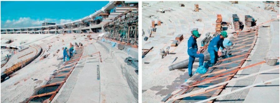
Figure 17.12 Strengthening the stadium tiers using carbon fiber TRM.
