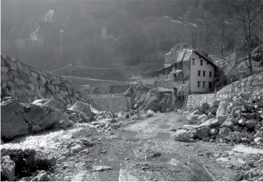
Figure 2. T. Lys (Gressoney, Italy), after the flood of 2002. Huge protection works along the banks are apparent, as is the dangerous proximity of the house to this aggressive water course (photo A. Goltara).
