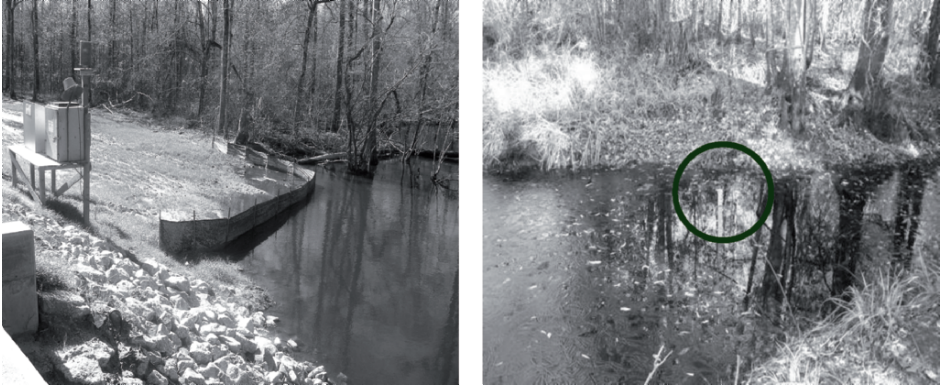
Figure 2. USGS real time precipitation and flow gauging station (# 02172035) downstream (left picture) and stage recording sensor (right picture) upstream of Highway 41 bridge at Turkey Creek watershed.
