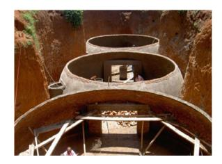
**Fig. 6.3** Internal baffle wall (Reprinted here with kind permission KfW 2009)
