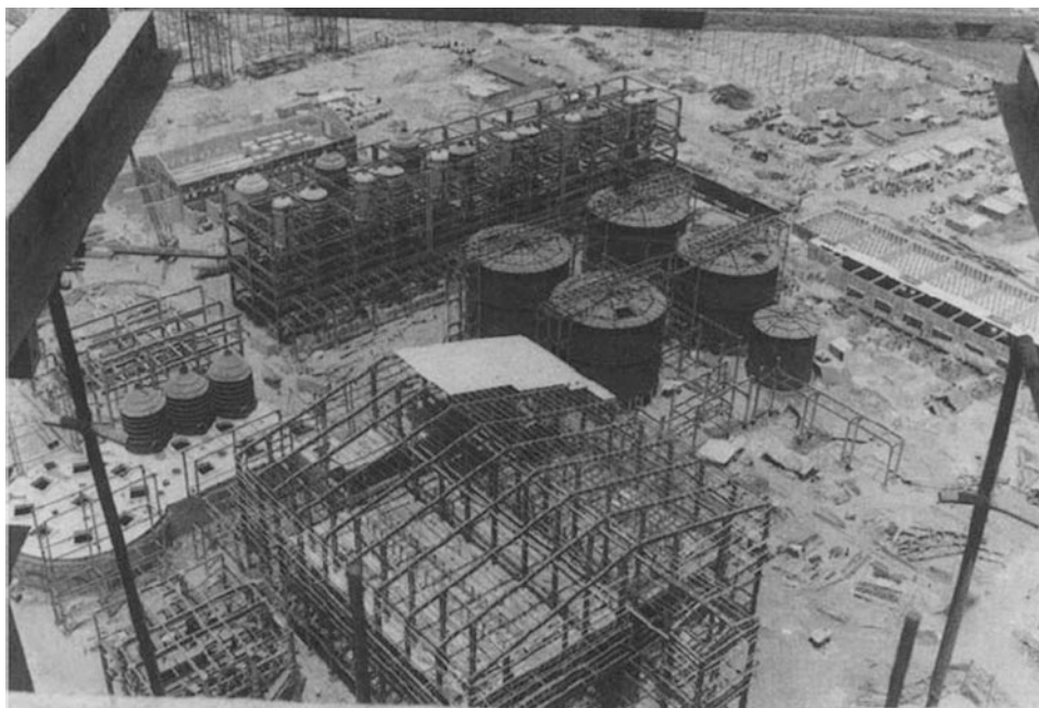
Fig. 23.10 Oswal phosphoric acid plant during construction—May 1999—Paradeep, Orissa, India
