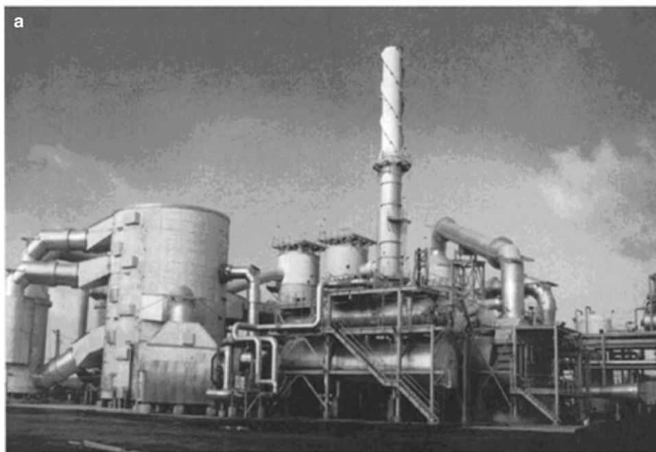
Fig. 25.6 (a) Modern double absorption sulfuric acid plant with view of sulfur furnace in foreground. (Courtesy Monsanto Enviro-Chem.). (b) Schematic flow diagram of a double absorption contact process for sulfuric acid manufacture
