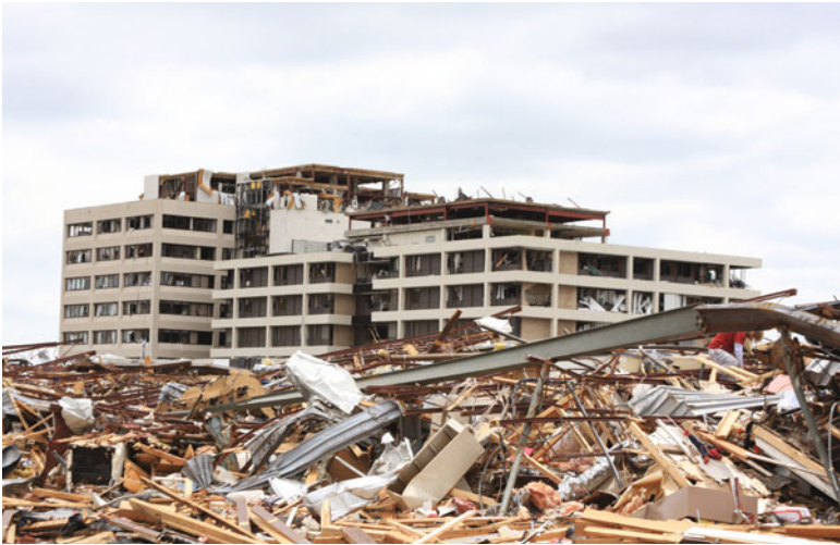
St. John's Mercy Hospital in Joplin, Missouri. Five patients and one visitor were killed when the tornado hit the building. The remaining structure is being demolished, while a new hospital is constructed 3 miles away.
