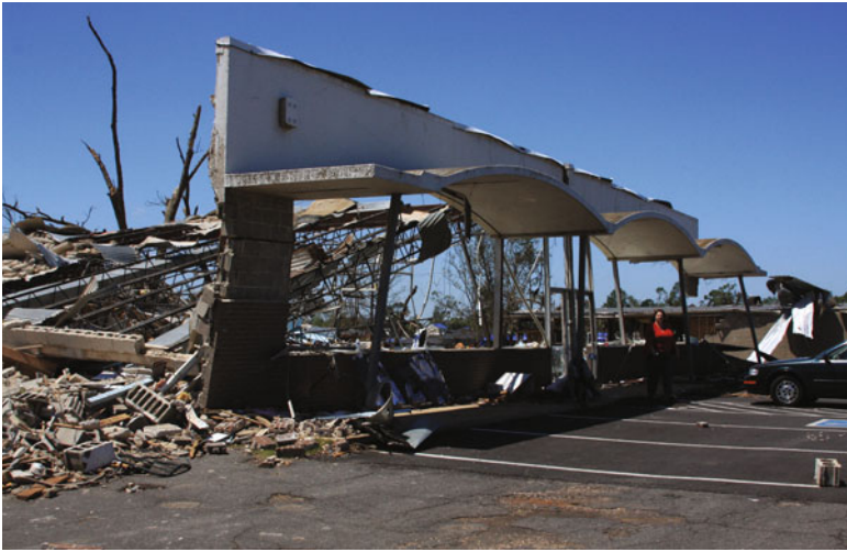
Commercial damage in Tuscaloosa, Alabama, from the April 27, 2011 tornado outbreak. Nearly 11,000 buildings were damaged in the EF-4 Tuscaloosa–Birmingham tornado.
