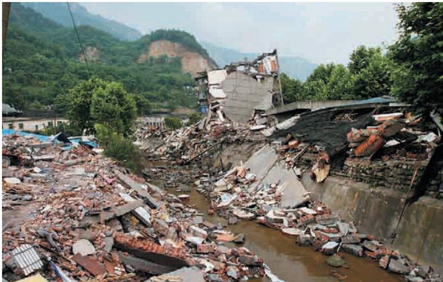
Figure 1.25 Complete collapse of old brick masonry house, Hanwang Village in Mianzhu City. Most village houses were built using experience rather than controlled professional design and construction. As a result, the earthquake caused massive destruction to these houses and enormous losses to life and property.
