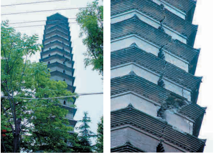
Figure 1.23 Most ancient structures in the earthquake affected areas had mortised timber frames, grey tiles, and brick or stone enclosure walls; most ancient pagodas were close-eaves brick pagodas. The main damage to ancient pagodas was cracking of the pagoda body and collapse at the top. The seventeen-storey Kuiguang pagoda in Dujiangyan City, a hexagonal brick tower, is shown. It shows cracking from top to bottom, and must be strengthened or repaired for further use.
