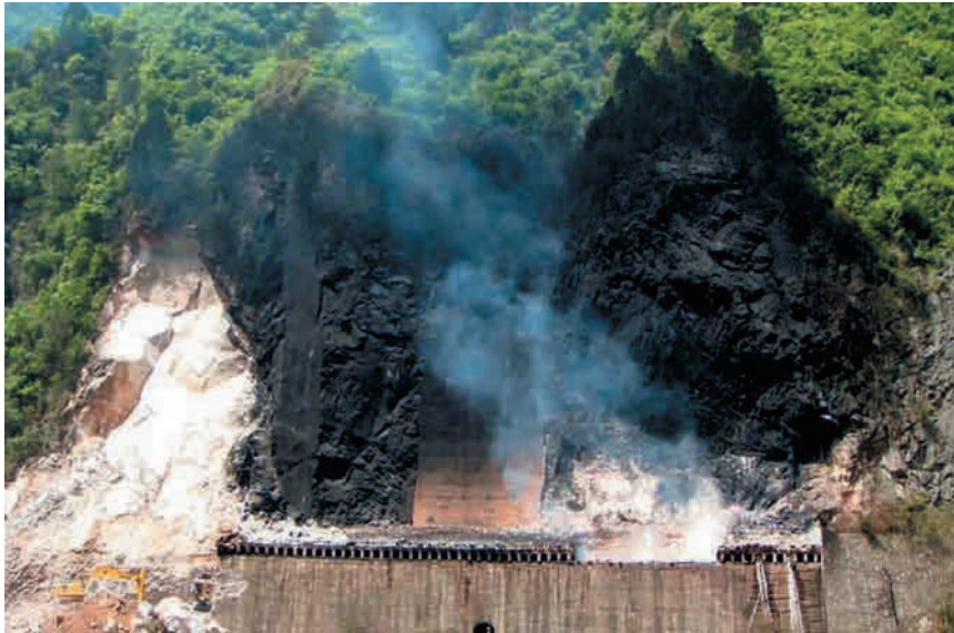
Figure 1.36 The most serious railway accident occurred at No. 109 tunnel on the Baoji–Chengdu line on 12 May. Large rocks falling from the mountain derailed a train of 40 gasoline trucks, blocked the tunnel, and caused an oilspill fire.
