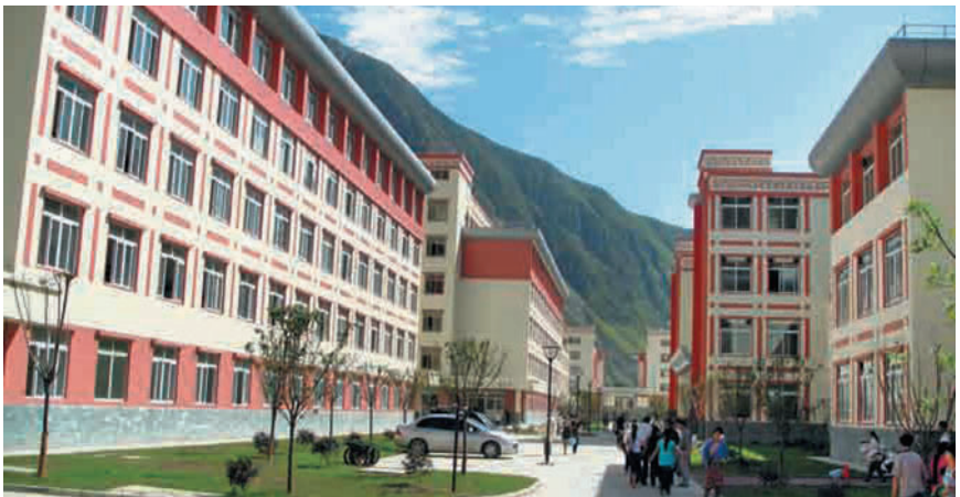
Figure 6.10 Buildings at the Wenchuan No. 2 Primary School compound in Sichuan Province have been rebuilt with new vibration-minimizing cushion technology (Photo by Dong Yong, Sichuan Earthquake Administration).
