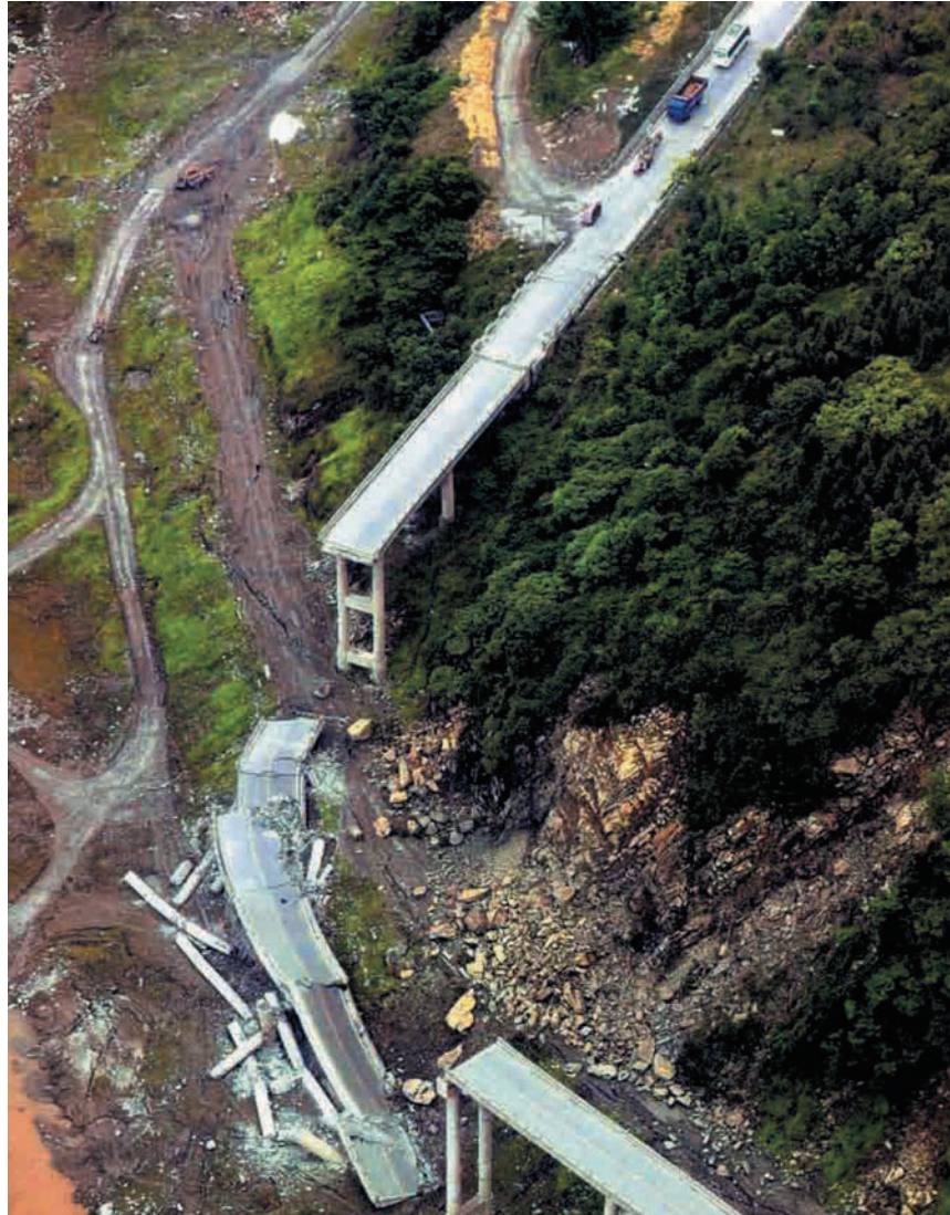
Figure 1.31 (a) Yingxiu bridge (Wenchuan County, intensity X), where a piece of bridge deck collapsed. Note: the rest stayed intact, with no damage (courtesy of Lu Ming). (b) The most severe damage to a highway bridge concerned the Baihua bridge collapse on the Dujiangyan to Yingxiu section of national road 213 (from “renmin” website).
