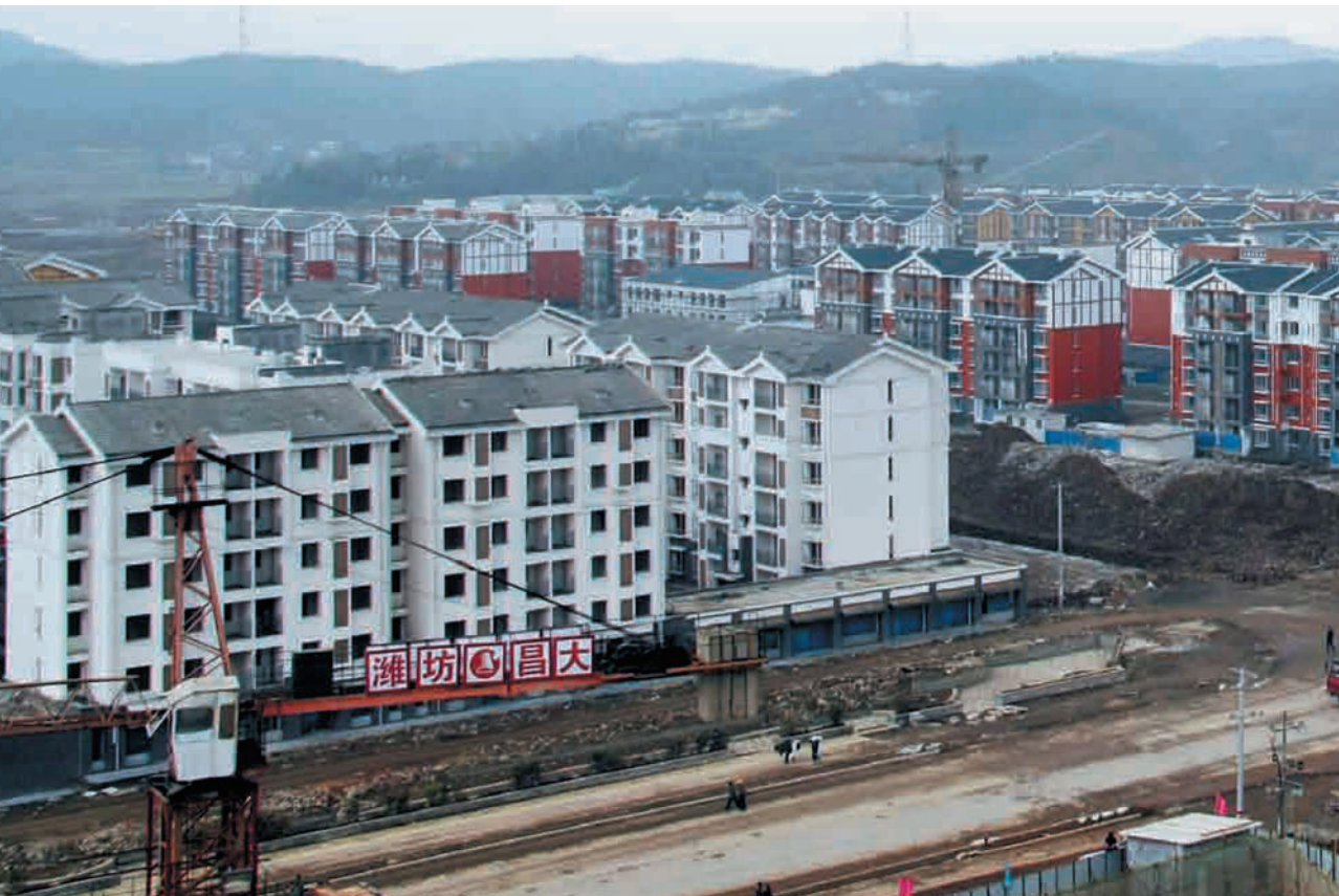
Figure 6.15 New housing in new Beichuan County, constructed by Shandong Province: 1.22 million m 2 11,084 homes.
