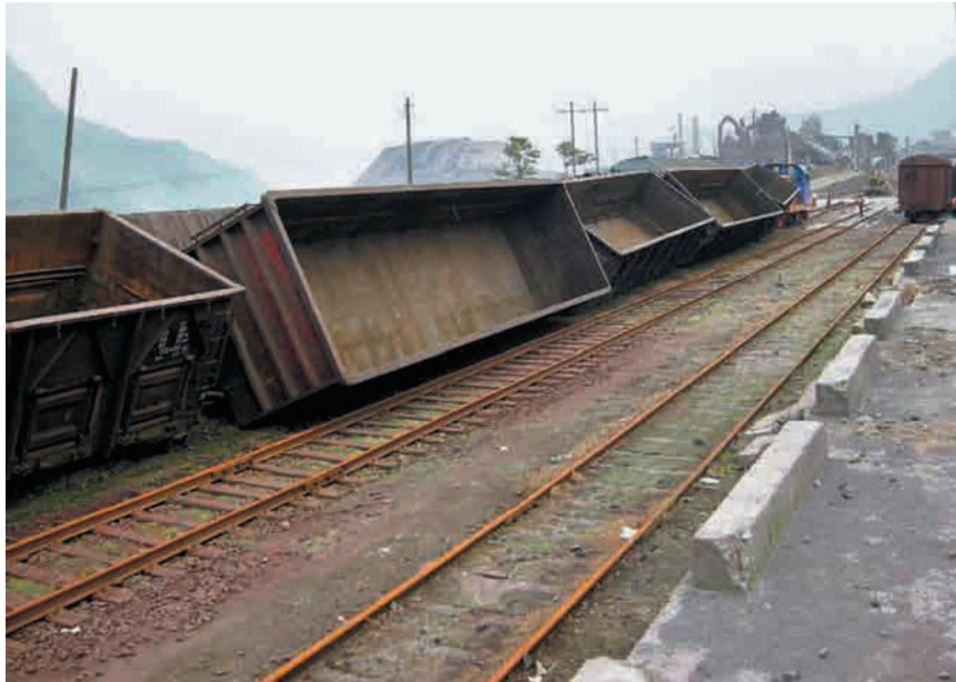
Figure 1.38 Strong ground shaking and deformed tracks caused train derailment.
