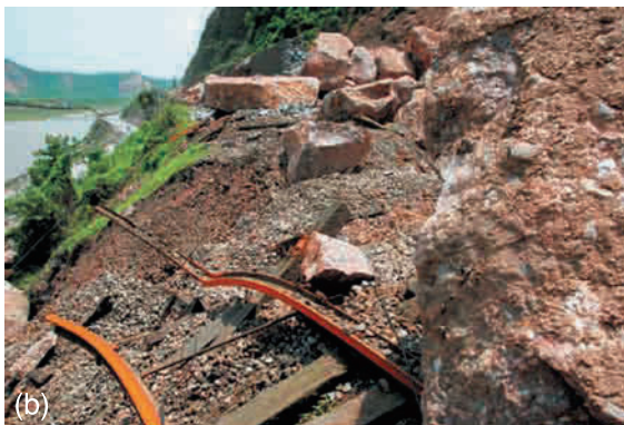
Figure 1.37 Damage to rails involved buckling and large deformation in either a vertical or horizontal direction. (a) Baoji–Chengdu railway line, Shifang section. (b) Railway line deformed by landslide, Shifang.
