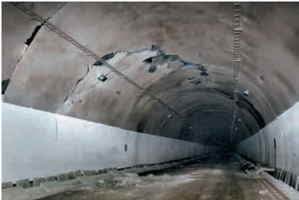
Figure 1.32 Damage at Longdongzi tunnel near Dujiangyan City, intensity X. The tunnel was visible damage to the film all the scenes. It is extremely rare during Wenchuan earthquake that fault through the tunnel, therefore, most of the tunnel (even in X degrees area) was slightly damaged, or no damage during earthquakes (courtesy of Lu Ming).
