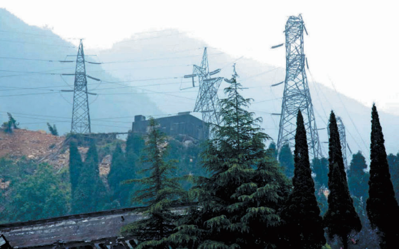
Figure 1.39 High voltage transmission line pylons toppled, Yingxiu Town in Wenchuan County.
