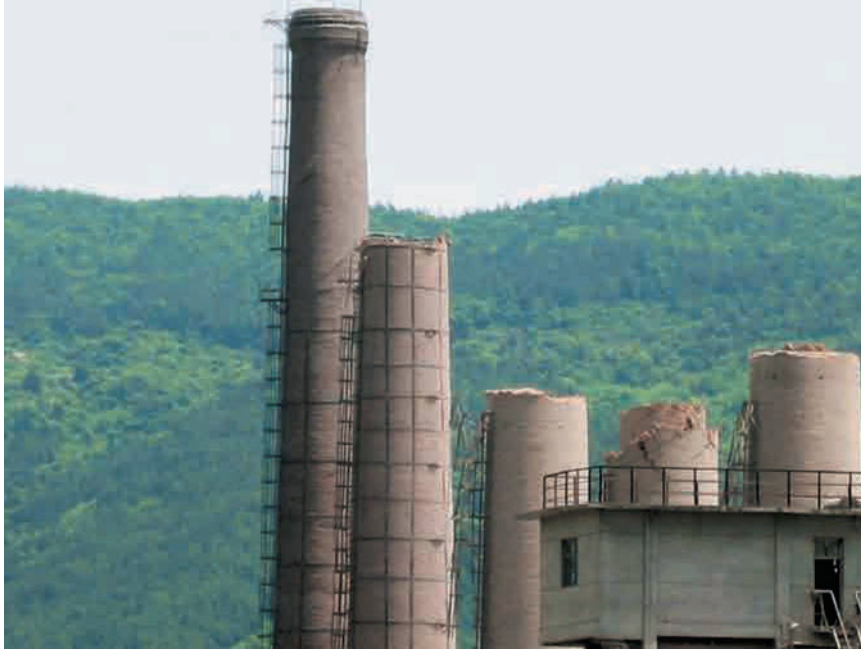
Figure 1.41 Jianguo Two-horse Group factory. Of five chimneys, four were decapitated.
