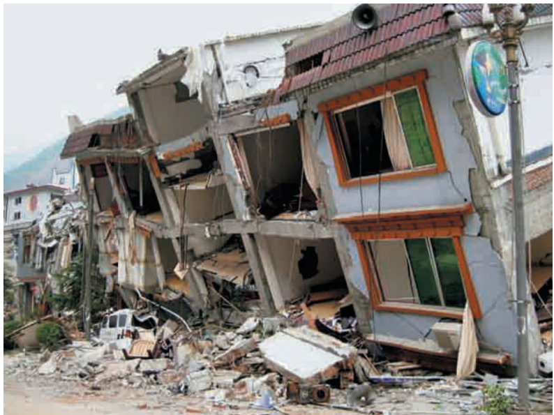
Figure 1.7 Total collapse of brick masonry residences in Yingxiu. (intensity XI)
