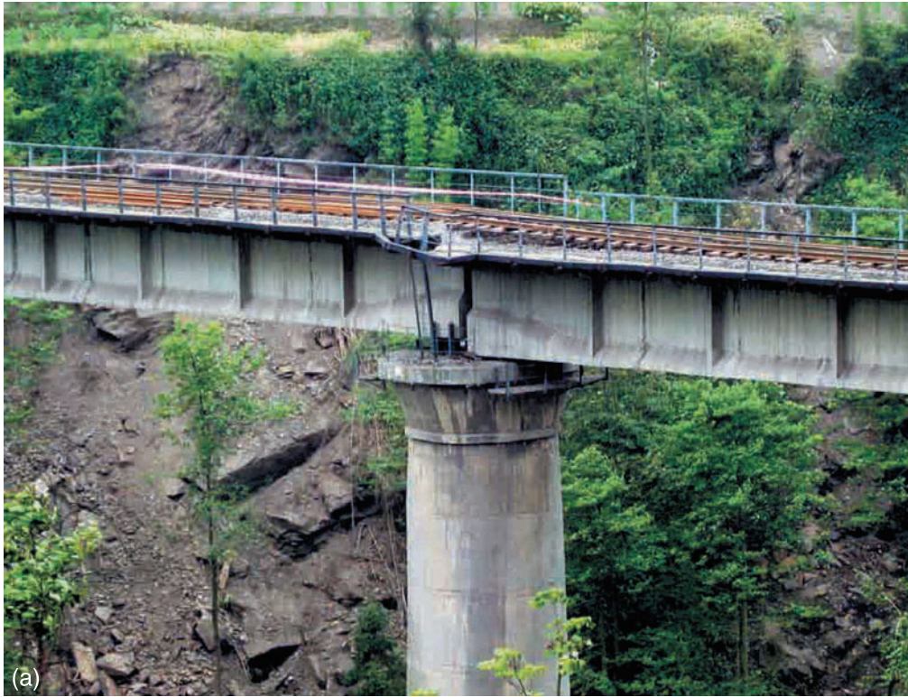
Figure 1.37 Damage to rails involved buckling and large deformation in either a vertical or horizontal direction. (a) Baoji–Chengdu railway line, Shifang section. (b) Railway line deformed by landslide, Shifang.
