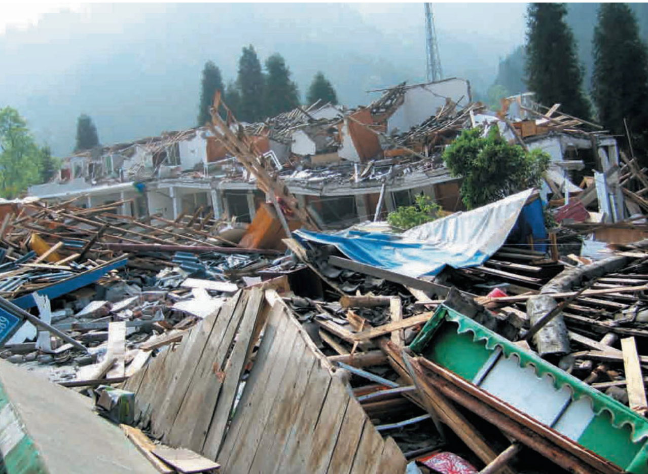
Figure 1.30 Rural residences, consisting mostly one- or two-storey masonry buildings, suffered much more extensive collapse than urban residences.
