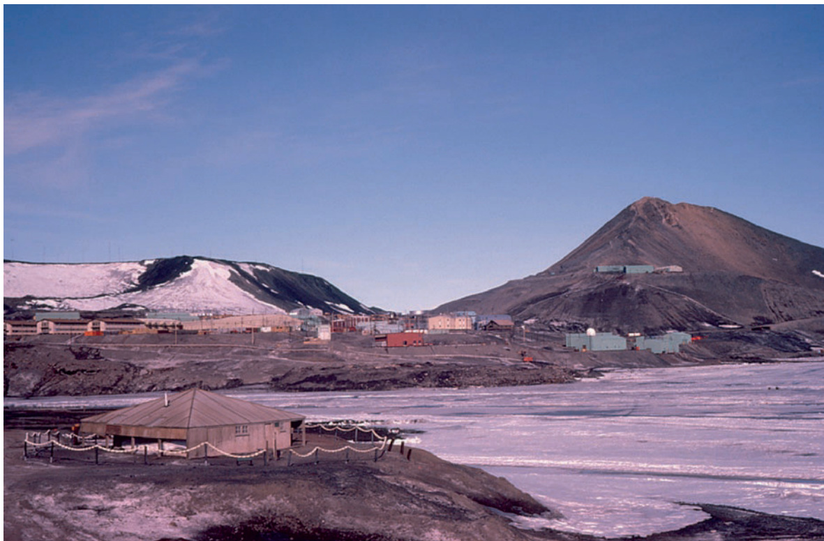
Fig. 2.9 View of McMurdo Station from Hut Point toward the Discovery Hut of Robert Scott (1901–1904) and Observation Hill in the background on the right. Arrival Heights is the basalt plateau on the left. The green building half-way up the slope of “Obs Hill” used to house the nuclear reactor that has since been
