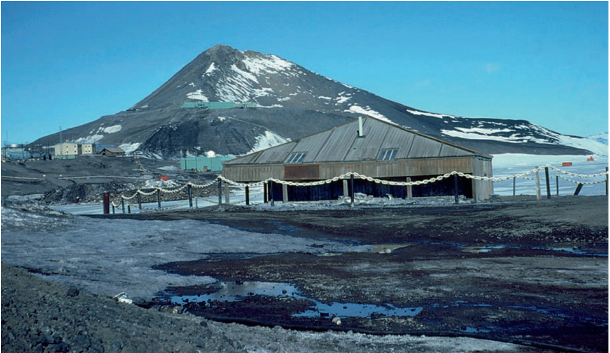
Fig. 1.10 The hut that Robert Scott and his men built in 1902 still stands at Hut Point where their ship, Discovery , was moored for two winters. The hut was not well-enough insulated to withstand the cold which forced the crew to live on the Discovery . Observation Hill looms in the background. The hut is on the list
