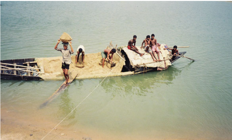
Plate 6.12 Riverbed sand quarrying from a boat at Majher Mana (1997 photo courtesy: Samir Ghosh)
