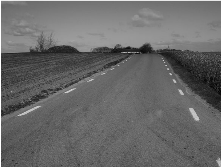
Fig. 13.2 Narrow roads and little space for equestrians in a typical Vellinge landscape (Photo: Courtesy of Daniel Melchert, God Bostad Kulturmiljökonsult)
