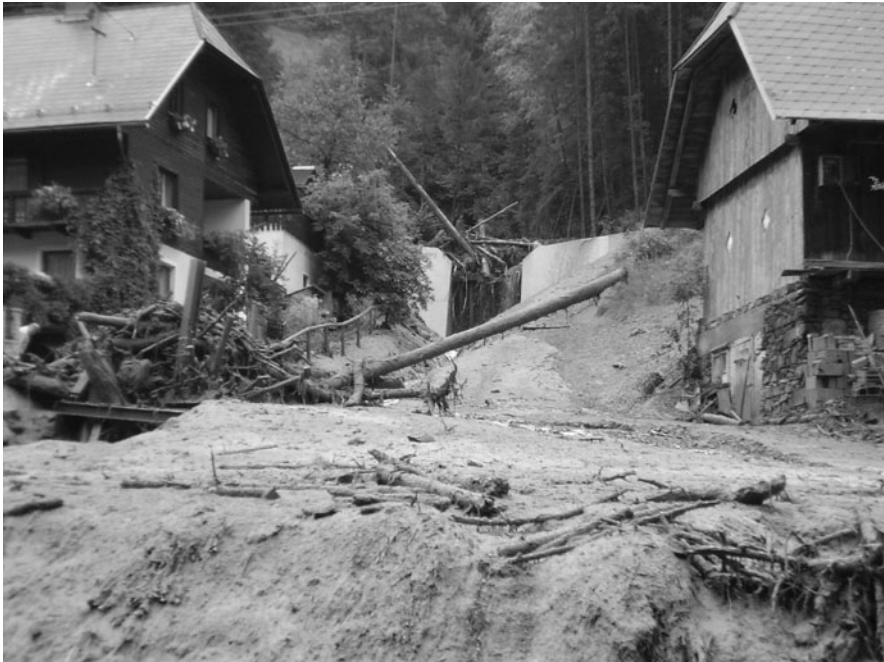
Fig. 3.3 Debris-sorting dam in the “Rauschergraben” (Community of Gasen, Austria). Impaired function and overload because of “Woody Debris”. Anyway, the measure could avoid heavy losses in the settlement (Photo: WLV Styria, Ellmer)
