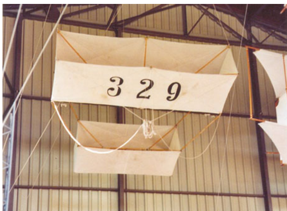
Fig. 1.1 Kite for atmospheric sounding from the beginning of the twentieth century at the Richard-Aßmann Observatory of the German Weather Service in Lindenberg (east of Berlin), Germany
