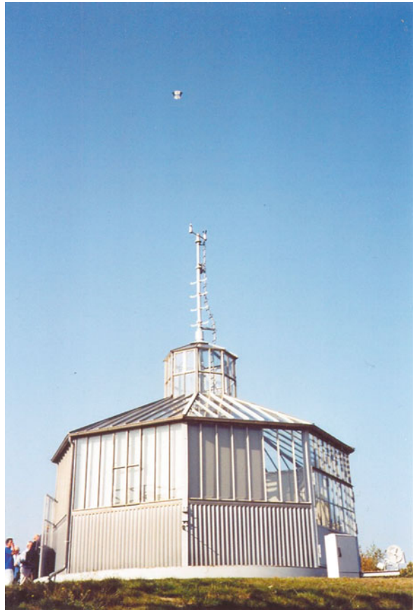
Fig. 1.2 Azimuthally turnable winch house at the Richard-Aßmann Observatory of the German Weather Service in Lindenberg (east of Berlin), Germany, built at the beginning of the twentieth century
