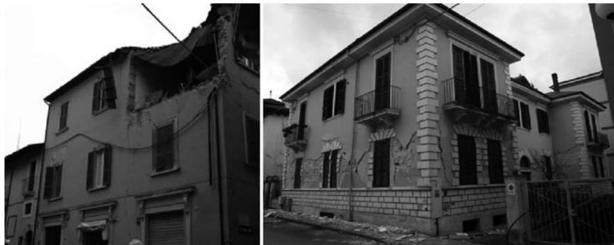
**Fig. 8.1** Examples of local out-of-plane failure mode (*left*) and global behavior, involving wall in-plane response (*right*), of masonry buildings during the 2009 Abruzzi earthquake in Italy
