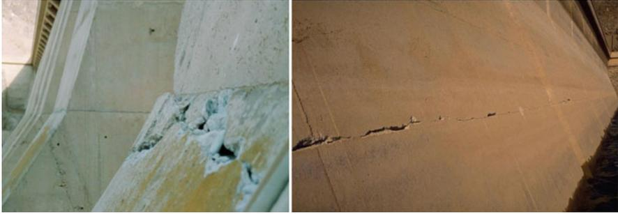
**Fig. 15.1** Cracks at downstream and upstream faces of Sefid Rud Dam (From Wieland 2009)
