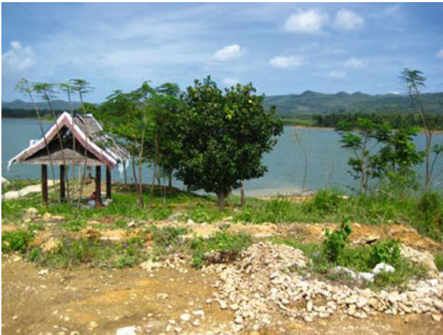
Fig. 2.10 A view of the reservoir of Malinao Dam in the municipality of Pilar, island province of Bohol. The dam is in the Wahig-Inabanga watershed and serves some 4,700 ha of ricelands
