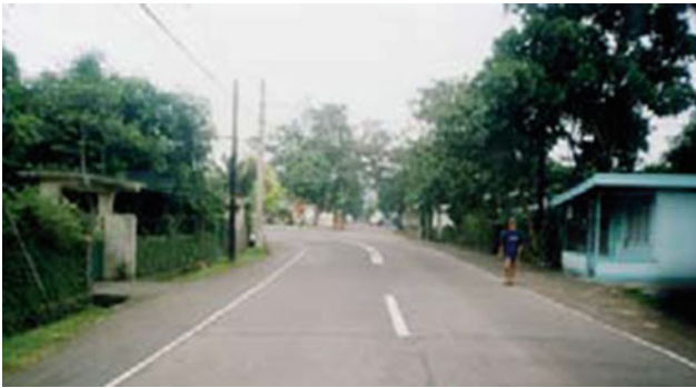
Fig. 5.2 As platform for human activities, our community life, especially our infrastructures relating to housing, transport, commerce, industry, and recreation stand on soils. With limited land resources, a major issue now is the competition for space between these different land uses
