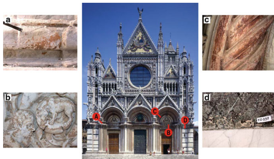
Fig. 1 Different types of Ca-oxalate films on the natural stone materials of the main façade of the Siena Cathedral: (a) and (b) on marble; (c) on red ammonitic limestone; (d) on serpentinite
