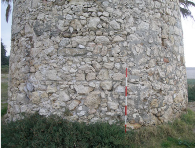
Fig. 1 Detail of the masonry, which highlights the “ cantiere ” technique
