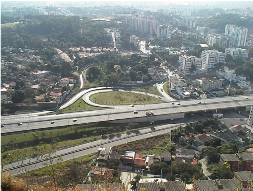
Fig. 3.16 Linha Amarela expressway (2003) (Photo: Author)
