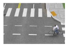
Intersection crossing markings or standard crosswalks can be used to highlight to cross traffic that bicyclists are crossing the roadway in that location. They may be used with crossing warning signs for bicycles or bicycles and pedestrians (MUTCD sign W11-1 or W11-15).
