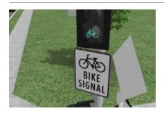
Bicycle signal heads can be added to a hybrid beacon to improve function and safety for bicyclists. See Bicycle Signal Heads for additional guidance.
