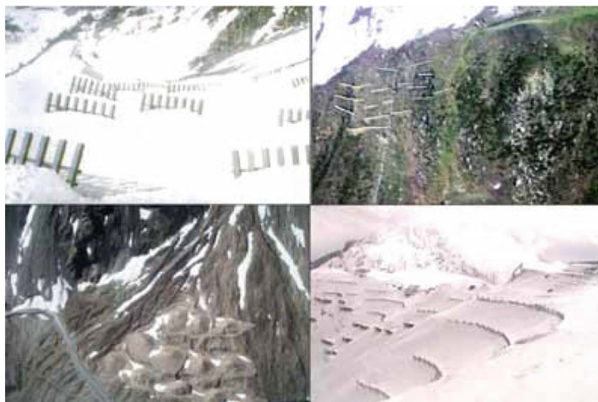
Fig. 1 Avalanche control structures for controlling avalanches and harvesting the Snow. Source Author
