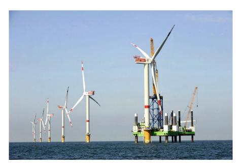
Fig. 3.9 Erecting an offshore array of REpower's 5-MW turbines (http://www.repower.de/)
