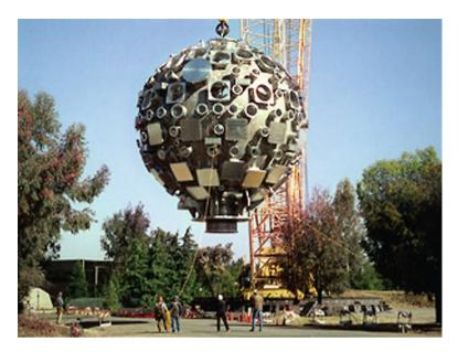
Fig. 10.51 The NIF target chamber being lifted into the building (https://www.llnl.gov/str/Atkinson.html.)
