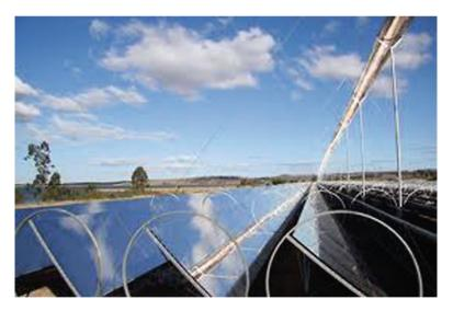
Fig. 3.27 A linear array of mirrors that rotate to follow the sun (http://www.instablogsimages. com/images/2007/09/21/ausra-solar-farm\_5810.jpg)
