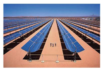
Fig. 3.26 A parabolic trough system (http://thoughtsonglobalwarming.blogspot.com/2008/03/ solar-thermal-company-says-it-could.html)
