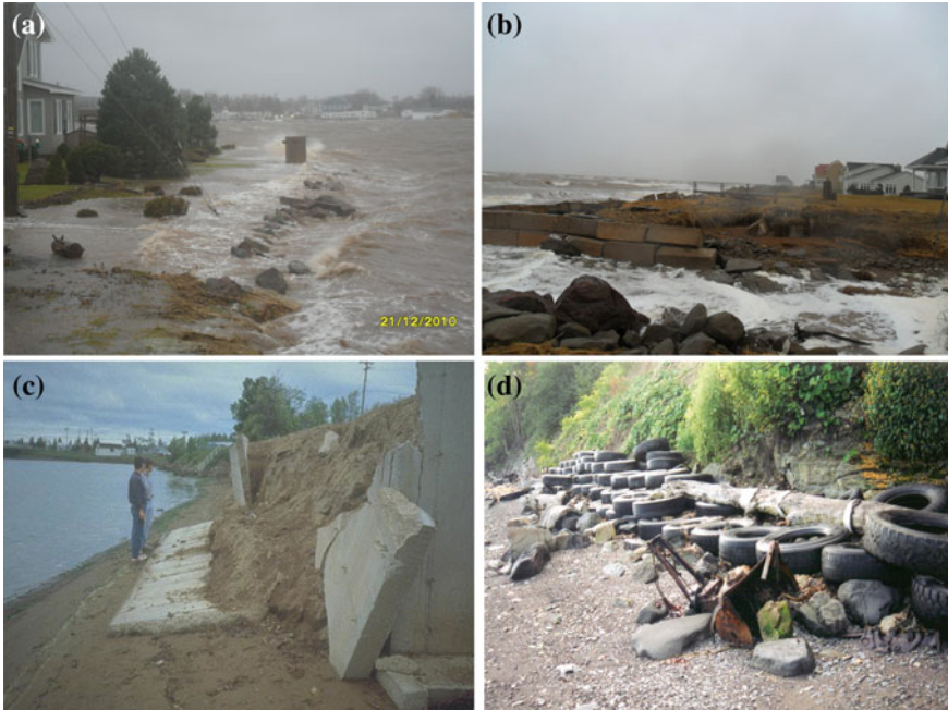
Fig. 3.5 Seawall failures: a overswept riff-raff seawall, b damaged brick seawall, c overtopped concrete seawall, d inefficient mixed material seawall in New Brunswick, Canada. Source (top) S. Doiron, 2010, ( bottom ) D. Bérubé, na
