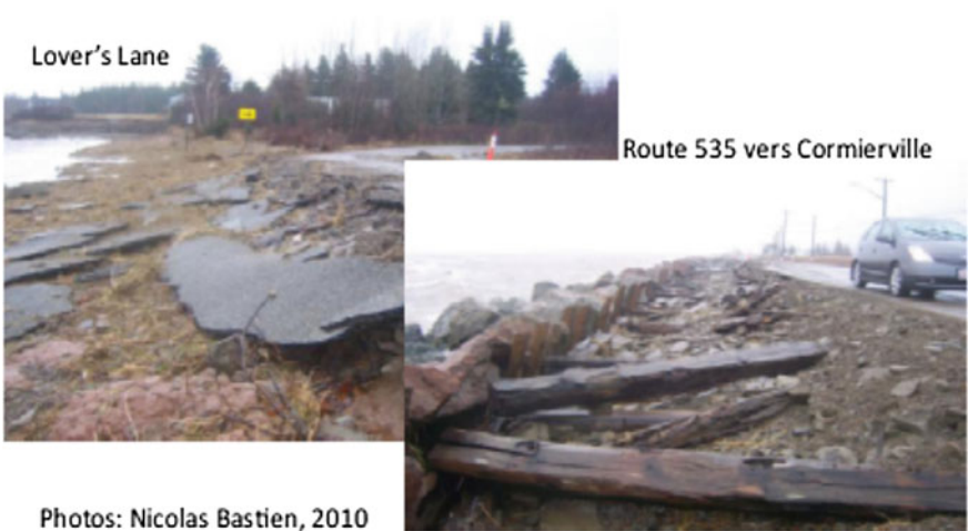
Fig. 4.10 Damages to local roads caused by the storm of 2010. Source N. Bastien, 2010
