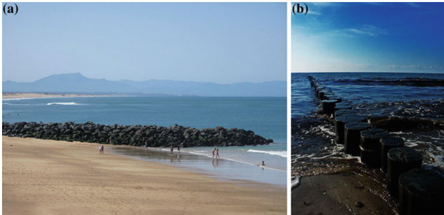
Fig. 3.9 Two different types of groynes, a stone groyne in Capbreton, Landes, France, b wooden piles in Markgrafenhede, Baltic Sea, Germany. Source a Tangopaso, 2009, in Wikipedia, b NiTen, 2006, in Wikipedia
