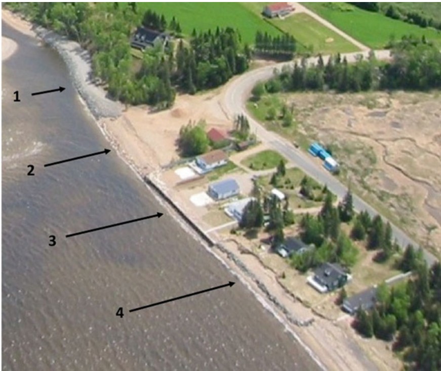
Fig. 4.4 Different types of protection structures at Carron Point: 1 heavy shale riff-raff, 2 small rock riff-raff, 3 cement wall, 4 large rock riff-raff. Source Chouinard et al. (2009a)
