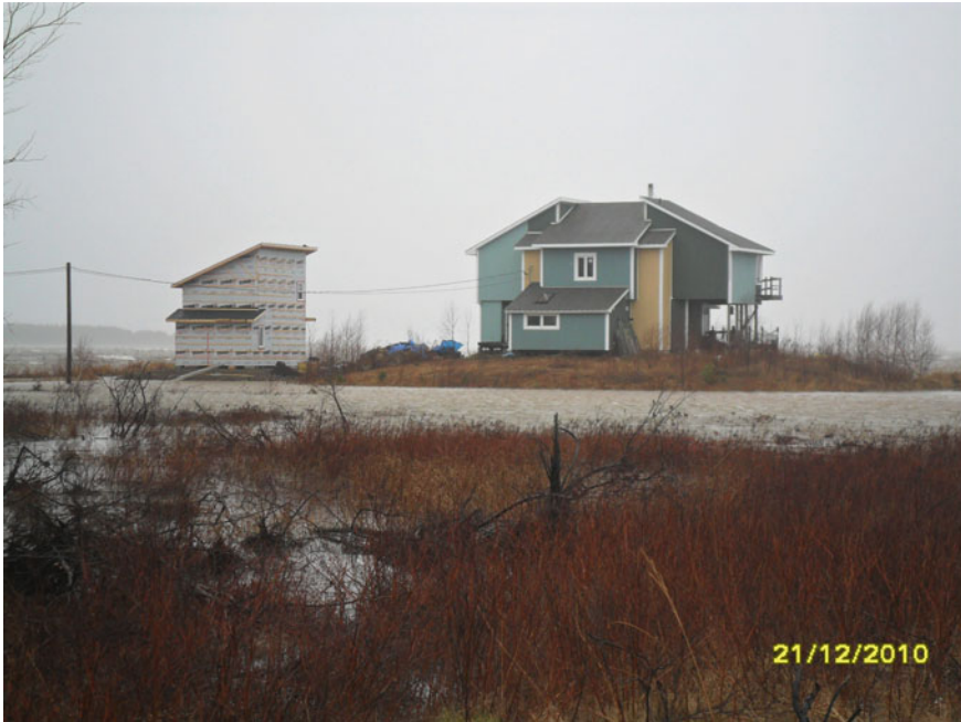
Fig. 3.13 House built on an artificial mound in the county of Westmorland, New Brunswick, Canada, surrounded by water during the flood of December 2010. Source S. Doiron, 2010
