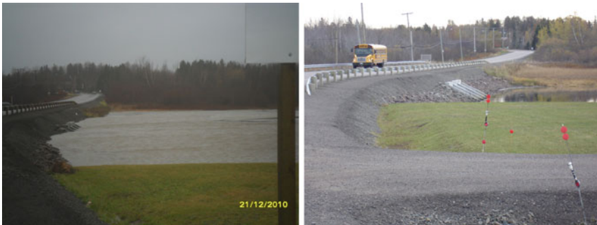
Fig. 4.13 The new bridge of Pointe-du-Chêne during the storm of 2010 and in normal weather. Source S. Doiron, 2010; S. Weissenberger, 2012
