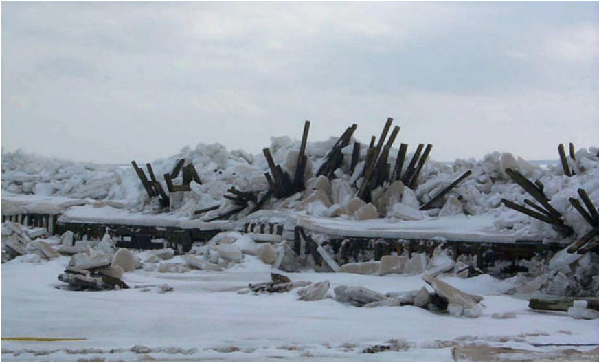
Fig. 4.9 Ice pile up on the Grande-Digue wharf in Cap-des-Caissie. Source Environment Canada, 2006
