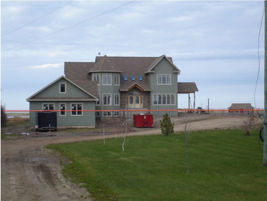
Fig. 3.15 House with living spaces above the maximum flood safety line in the county of Westmorland, New Brunswick, Canada. Source S. Weissenberger, 2012
