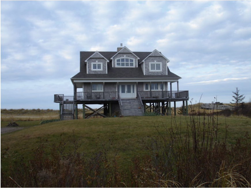
Fig. 3.14 House built on stilts in the county of Westmorland, New Brunswick, Canada. Source S. Weissenberger, 2012
