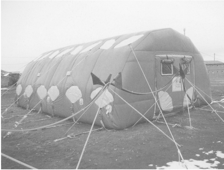
Fig. 2.9 This inflatable building was tested by NASA in Antarctica to determine if it could someday be used on the Moon. NASA's Innovative Partnership Program investigated using inflatable structures for future long-term lunar habitats. Weighing less than 1,000 pounds, the building inflates in fewer than 10 minutes. This photo was taken at McMurdo Station. (Courtesy NASA)
