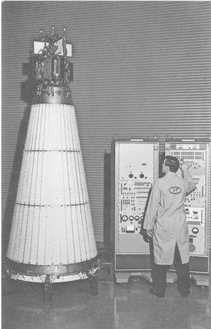
Fig. 9.6 The world's first nuclear reactor power plant to operate in space, SNAP-10A, was launched into Earth orbit on 3 April 1965. (Courtesy U.S. Department of Energy)
