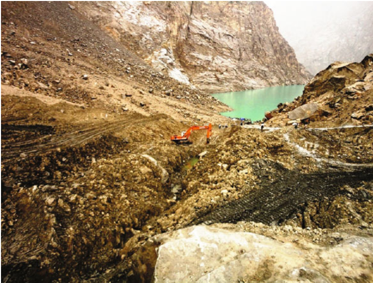
Fig. 1.24 Excavation of spillway in the debris of the Attabad rockslide dam, Hunza valley, northern Pakistan. The Hunza rockslide dammed lake is visible in the background. Photograph taken on April 18 (Day 102 of impoundment) when the lake level was at about 2,405 m a.s.l., 30 m below the eventual overflow elevation ( Pamir Times photograph)
