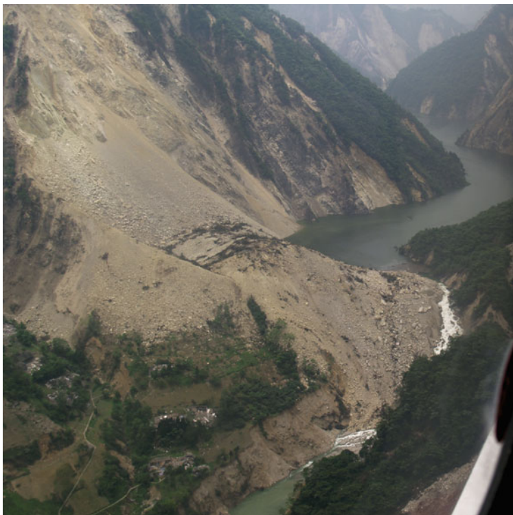
Fig. 10.16 Aerial view of Xiaogangjian #1 rockslide dam. View is upstream
