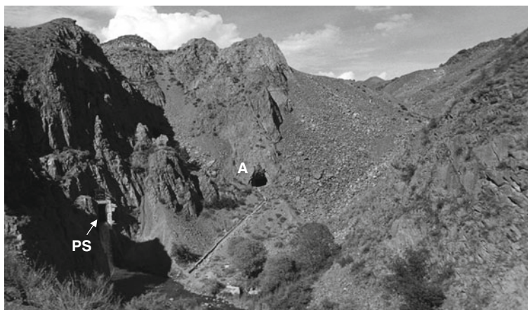
Fig. 26.1 The Burlykia experimental blast-fill dam. A – adit at the base of the right slope that was made to investigate seismic effect of the explosion on the underground structures. PS – permanent spillway. View from downstream
