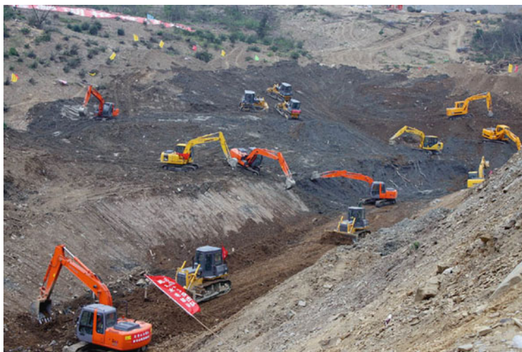
Fig. 10.11 The Tangjiashan sluiceway under construction (Provided by Water Resources Bureau of Mianyang city)
