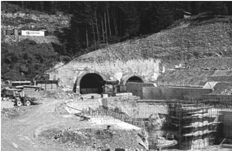
Fig. 2.13 Exit portals for the twin-bore diversion tunnel that carries the Adda River around the Val Pola landslide dam. The tunnel on the right was operational at the time of the photo, and the left-hand tunnel was near completion
