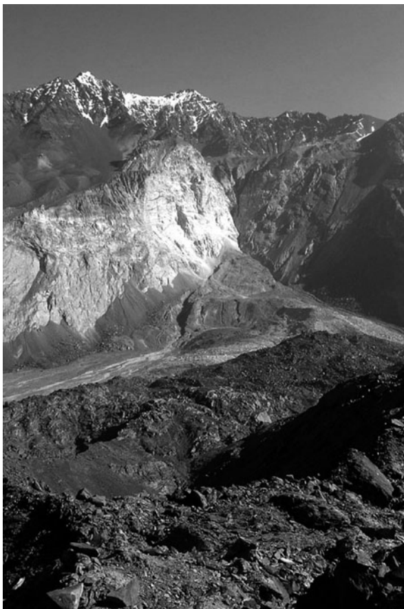
Fig. 16.5 Helicopter view of the scarp of the Usoi landslide from the highest point of the dam (photo A. Ischuk, 2004)
