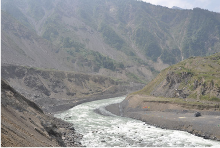
Fig. 10.15 Tangjiashan Lake: upstream view of the armoured spillway channel bed 15 months after risk reduction operation (Photograph taken on September 22, 2009)
