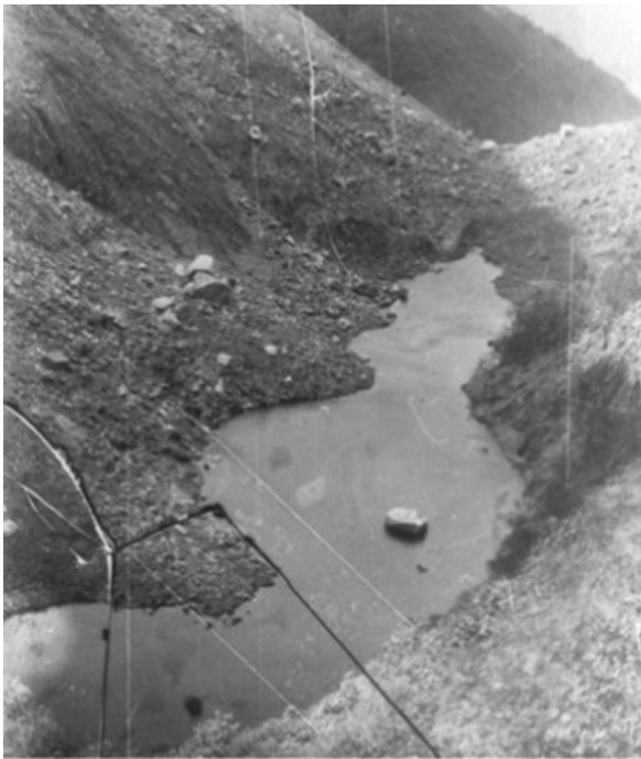
Fig. 3.8 View of the Motto d'Arbino rockfall dam in the Arbedo Valley, taken just after the event, in 1928
