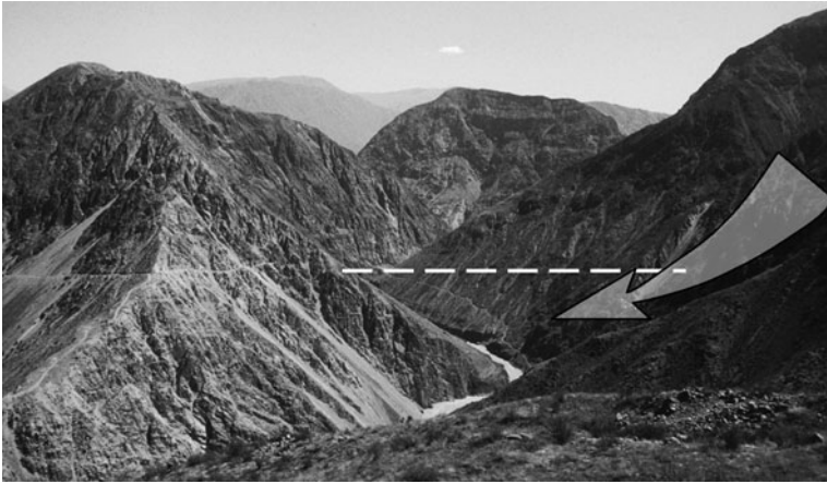
Fig. 25.20 The Kambarata-1 dam site. Dashed line corresponds to the designed dam crest; arrow shows the direction of rock sliding
