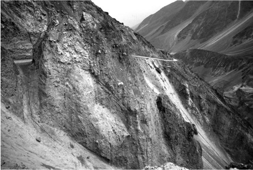
Fig. 6.11 Mountain road cut through a rock avalanche, the Bilchar event, in Bagrot valley, Gilgit District. The vertical cuts testify to the strength and compaction of the rock avalanche material, but rainfall and snowmelt can generate sudden collapses or debris flows at the surface. The landslide once formed a dam on the Bagrot River [28]
