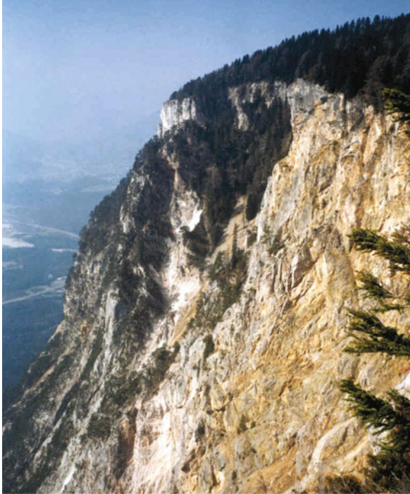
Fig. 3.3 View of the top scarp of the Dobratsch rockslide. Large fissures can be seen in the forest on the top
