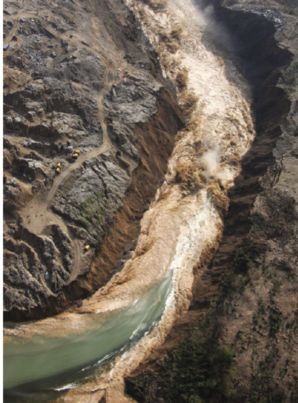
Fig. 1.22 Aerial view of flow in Tangjiashan spillway at about 9 a.m. June 10, 2008, during controlled partial drainage/breaching of rockslide dam. Discharge is approximately 2,000 \text{ m}^3/\text{s} . Note effects of spillway erosion and construction machinery for scale (photograph by Xinhua News Agency, China)
