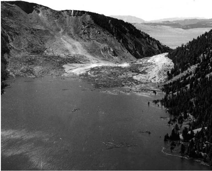
Fig. 1.2 Rockslide-dammed lake (Earthquake Lake) formed by landslide (est. vol. 20 \text{ Mm}^3 ) triggered by the M7.3 Hegben Lake earthquake, Montana, USA, August 17, 1959. Maximum volume of Earthquake Lake was 102 \text{ Mm}^3 [269]. Photograph was taken after construction of spillway (visible as a light area in the low centre of the debris) had begun (USGS photograph by John R. Stacy)
