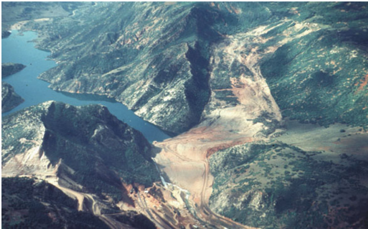
Fig. 2.9 The 1983 Thistle debris slide and its temporary impoundment, Thistle Lake. The lake was drained by a tunnel constructed through the mountain at the lower left
