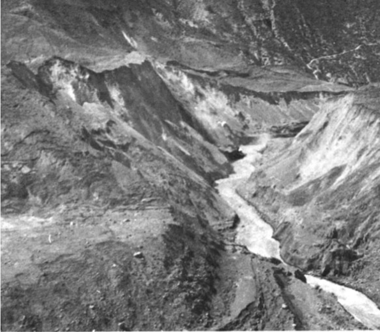
Fig. 3.14 Erosion gorge in the Mayunmarca Landslide dam after the outflow, more than 100 m deep
