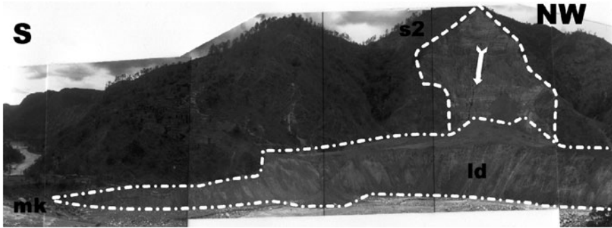
Fig. 8.26 Panoramic view over the remnants of DhARBANG landslide dam ( ld ): Note the morphology of the cone of landslide debris); s2 = scarp (1988), ↓ = direction of movement, mk = Myagdi Khola River
