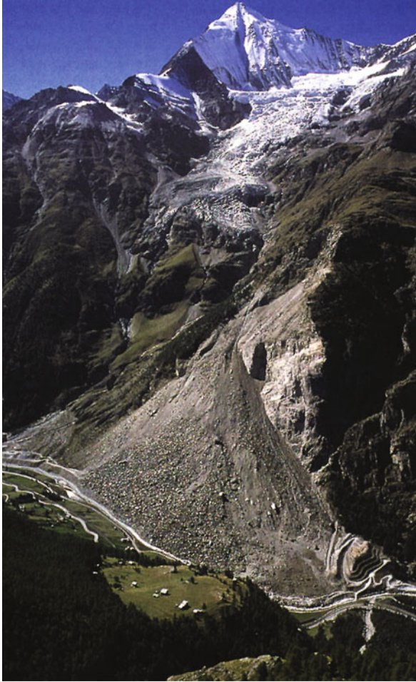
Fig. 3.11 General view of the Randa rockfall causing the damming of the Vispa River. The mitigation works have been already carried out
