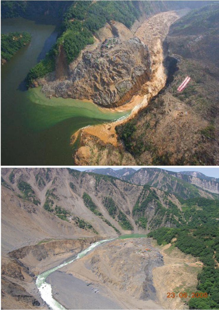
Fig. 10.14 Tangjiashan rockslide-dammed lake during and after partial drainage on June 10, 2008. Upper picture (view downstream) shows the incised channel over the debris caused by water release from Tangjiashan lake through the sluiceway (photograph from Prof. Liu Ning). Lower photograph (view upstream) is an overview of new channel after water release from Tangjiashan landslide lake (photograph is provided by Water Resources Bureau of Mianyang city)
