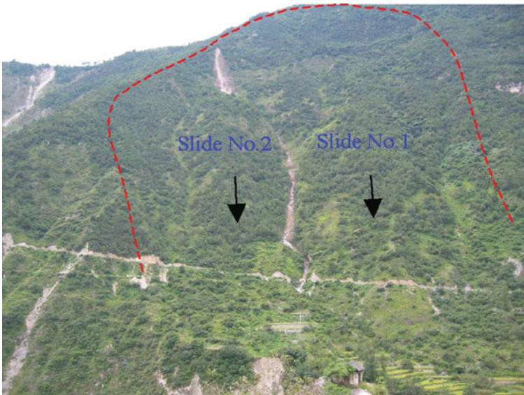
Fig. 13.6 Photograph showing the landslide site (view is to the west). The failure main scarp is marked with a dashed line and the location of the site shown in Fig. 13.4
