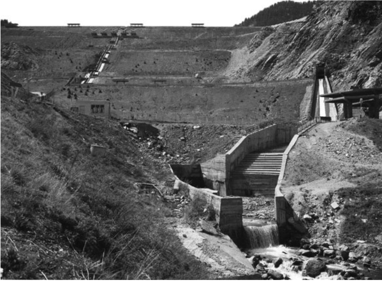
Fig. 1.30 View upstream of the Medeo debris retention dam constructed in multiple phases between 1966 and 1975 on the Malaya Almaatinka River, Zailiysky Alatau Mountains, Kazakhstan. The present debris flow retention capacity of the structure is 12.6 \text{ Mm}^3 . Note the bypass tunnel and spillway at the right of the photograph designed to drain water content of debris flows through the dam to the downstream channel (reproduced from High Dams of the USSR , Technopromexport, 1989)
