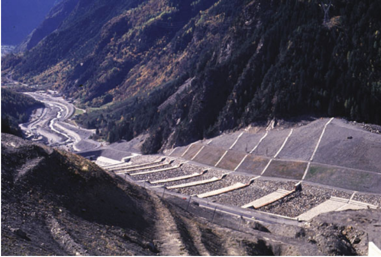
Fig. 2.12 Open-channel spillway, concrete sills, and a check dam under construction on the downstream slope of the Val Pola landslide dam
