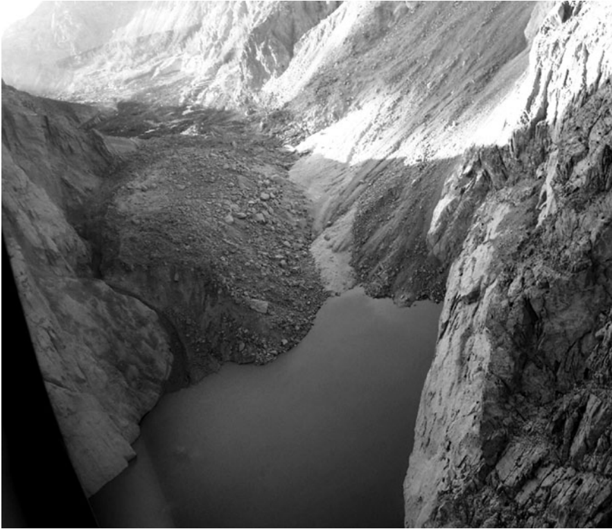
Fig. 7.11 Aerial view of Attabad rockslide (est. vol. 55 \text{ Mm}^3 ) that blocked the Hunza River, northern Pakistan on January 4, 2010. Rockslide slid from right. Rockslide-dammed lake is filling behind the debris on January 17 (Day 13 of impoundment). View is downstream. [ Pamir Times photograph]
