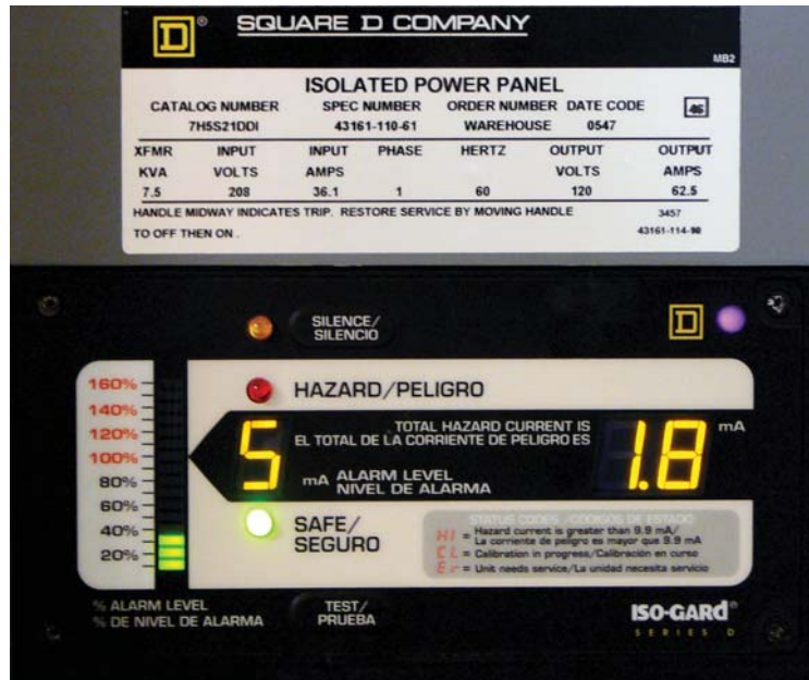
FIGURE 27-12. A. Isolated-power system. Note that neither side of the secondary of the transformer is connected to ground terminals, either at the transformer or at the circuit breaker box. B. Old and new (digital) line-isolation monitor status indicators. Digital panel indicates a total hazard current of 1.8 mA.
