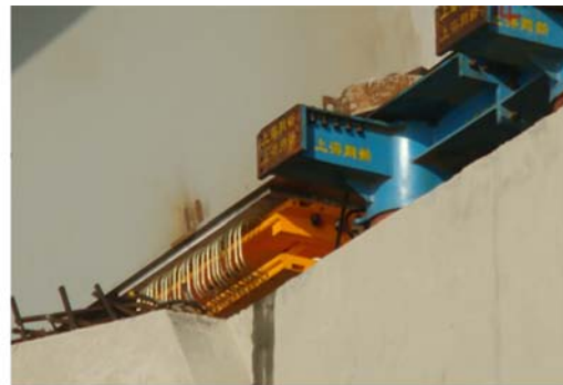
(b) Site installation of the bearing
