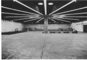
Figure 5.2 Kensington & Chelsea Maintenance Depot. (Arup Associates, Architects, Engineers & Quantity Surveyors.)
