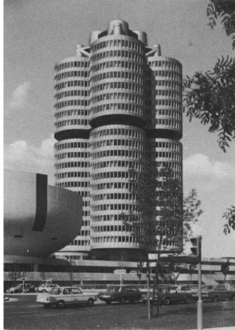
Figure 7.12 BMW Central Administration Building, Munich.
