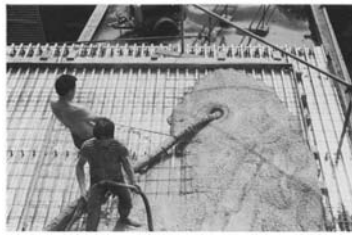
Figure 4.3 Pumped lightweight aggregate concrete being placed on metal decking.
