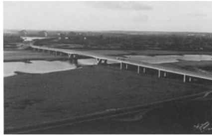
Figure 6.7 Completed Koningspleijbrug (photo: Aerofoto Brouwer-Brummen).
