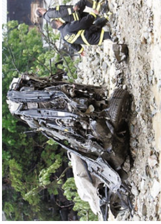
Fig. 7.3. Damage to infrastructures in the Val Chisone, Italy, flash flood 2008
