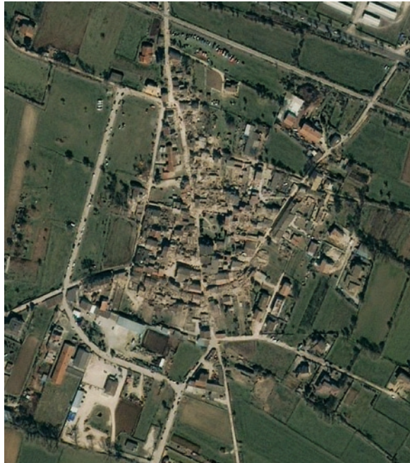
Fig. 17.7 Onna aerial view showing the damage to the building stock
