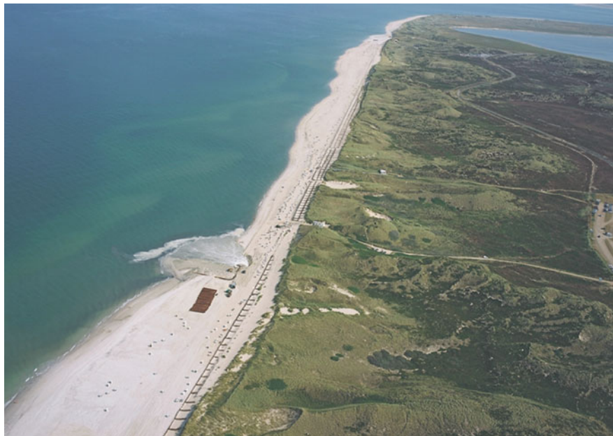
Fig. 6.6 Sand replenishment on the beach of the Isle of Sylt (Germany)
