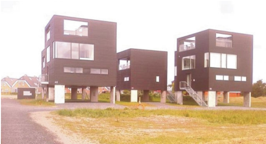
Fig. 6.5 Summerhouses on stilts in a flood-prone lowland on the Isle of Rømø (Denmark)
