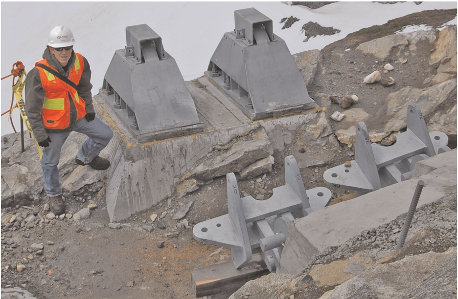
Figure 6.15 Cable anchorage yoke plates and saddles
