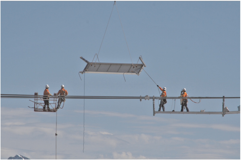
Figure 6.10 Dropping in a catwalk section by helicopter
