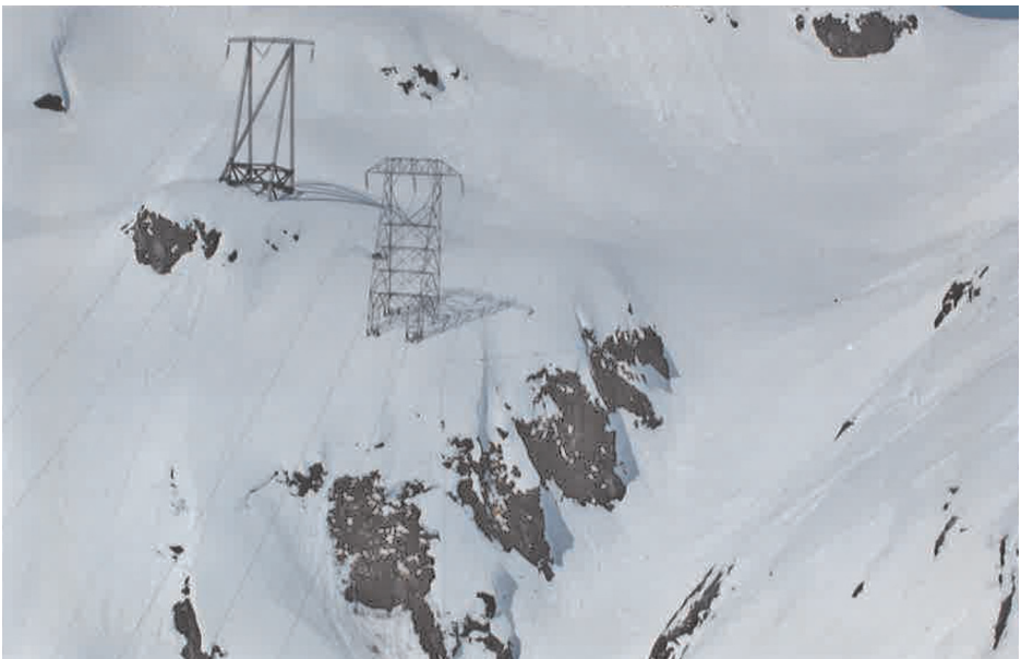
Figure 7.6 Tower 113R in the foreground and tower 114L behind it
