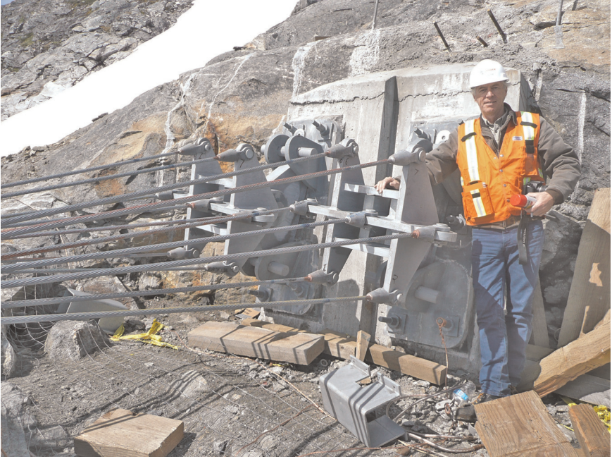
Figure 6.14 The author with the yoke plates of the vertical anchorage design
