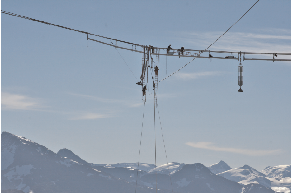
Figure 6.13 Hanging the first phase from Cat 2. (Courtesy of Erik Ruggeri)
