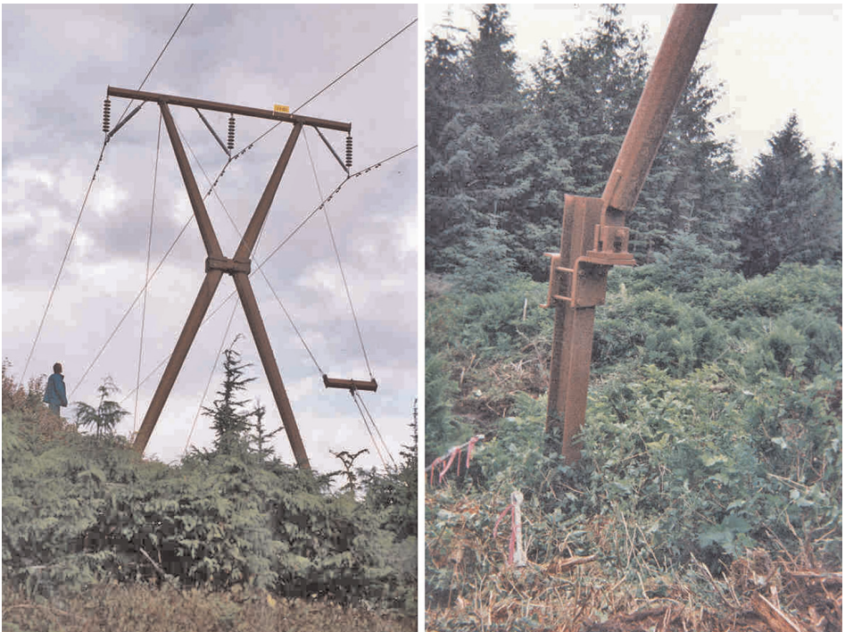
Figure 7.11 The tubular X tower (138 kV), Alaska
