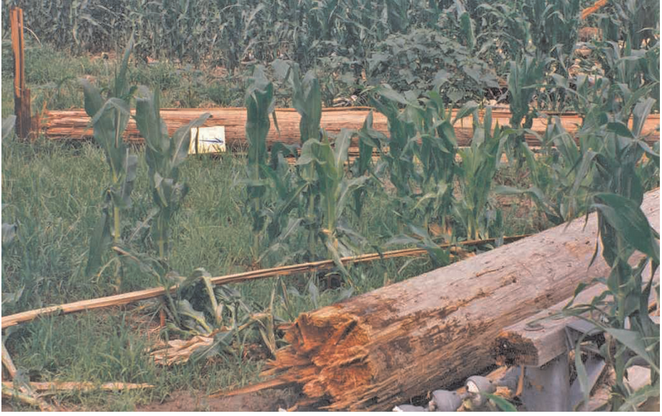
Figure 7.1 Radial knots at the ground line of the first pole to fail
