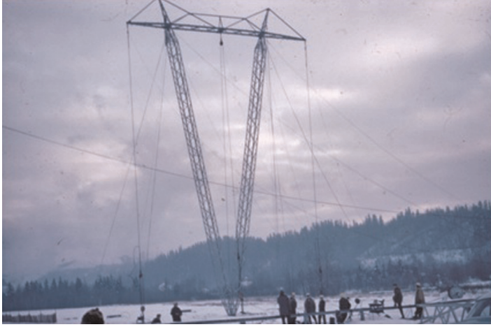
Figure 4.8 A first-generation 345 kV guyed-V tower. (Courtesy of H. Brian White)
