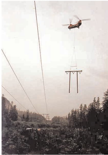
Figure 7.12 Flying the guyed-V tower into the existing line
