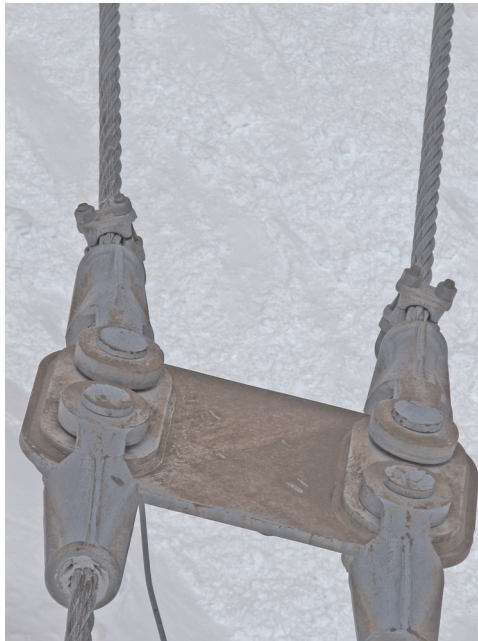
Figure 6.4 Catenary 1 yoke plate at the catwalk ends
