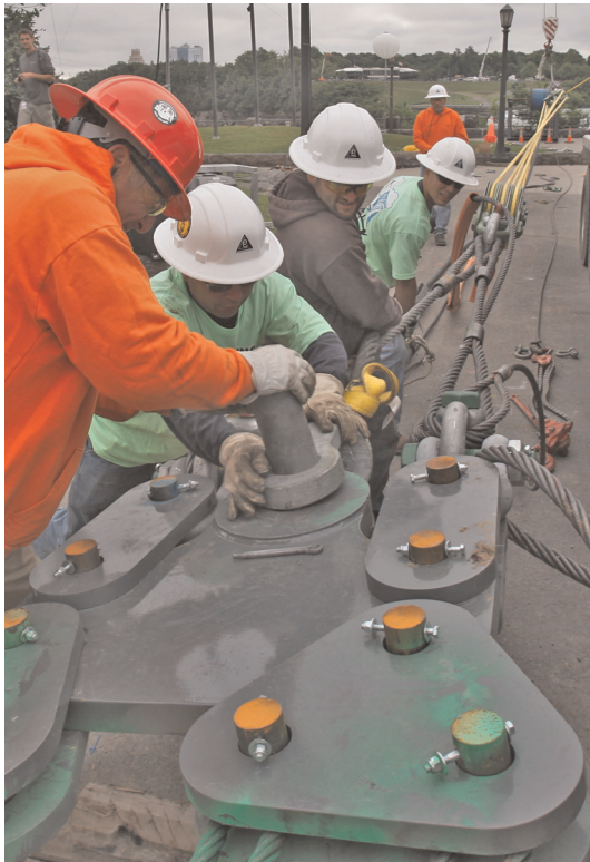
Figure 6.17 Pinning the cable to the yoke plate. (Courtesy of Steve Behal)
