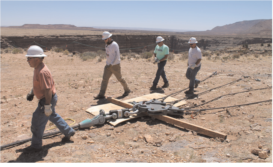
Figure 6.19 Four anchors and cables yoked to the walking cable
