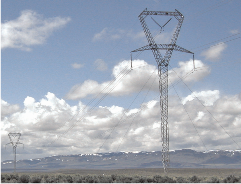
Figure 4.12 A single-circuit 345 kV gayed 'banjo' tower. (Courtesy of POWER Engineers)
