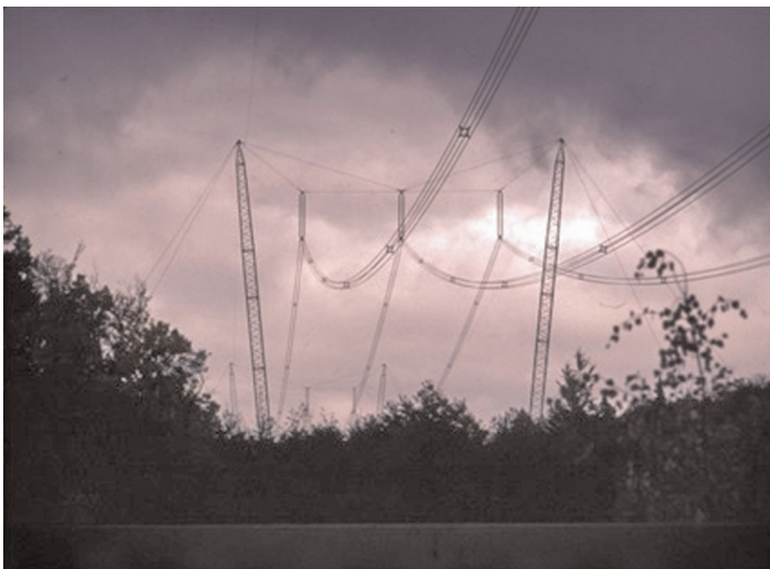
Figure 4.9 A 735 kV CRS design. (Courtesy of H. Brian White)
