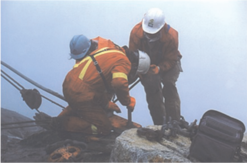
Figure 7.8 Pinning the temporary catenary to the temporary anchor
