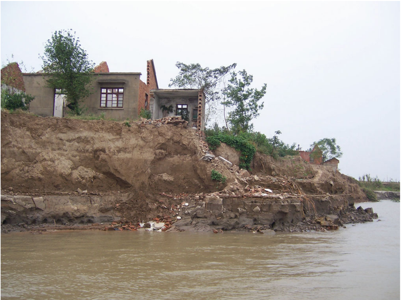
Photo 1.2 In the middle and lower reaches of the Changjiang, the river travels over fluvial plains with a width of several kilometers. Floods can cause the erosion of shoals in this region and damage to
