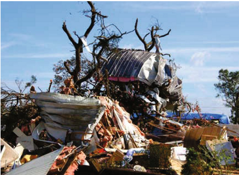
Mobile home damage due to tornadic winds.
