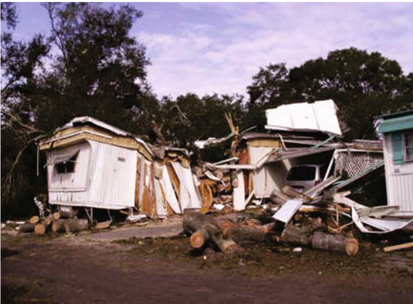
February 2, 2007: Typical tree damage to homes in Sunshine Mobile Home Park, Lady Lake, Florida, caused by EF-3 tornadic winds of 150 mph. This mobile home park consisted of mostly older units, built in the 1970s and '80s. Because the homes were pre-1994, tie downs were sparse or widely spaced. Many of the tie downs were rusted near the ground and failed along the rusted sections.
