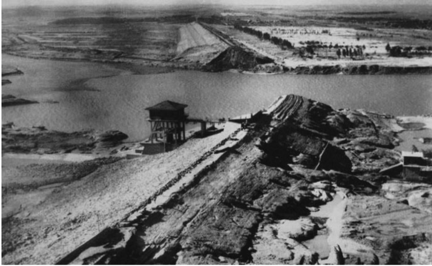
Fig. 33.1 The flood caused by the great storm of 75.8 in Henan destroyed the dam of the Banqiao reservoir
