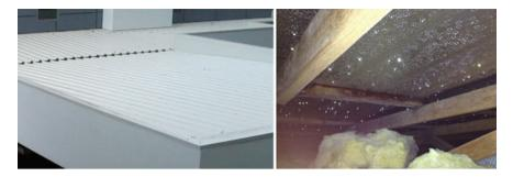
Fig. 13 The constantly wet, and often dripping underside of the roof
