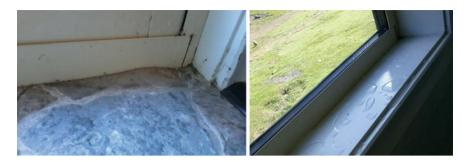
Fig. 19 Condensation forming on the kitchen flooring due to poorly installed insulation and a vapour impermeable vinyl finish. Around the window reveals the thermal bridging of the structure results in condensation
