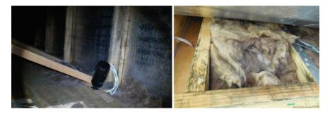
Fig. 21 Under the bed, the wall and carpet have limited exposure to the heating and experience thermal bridging to the external walls
