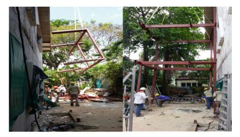
Fig. 5 Lifting and installing onto pre-fixed sleeves of first module on site
