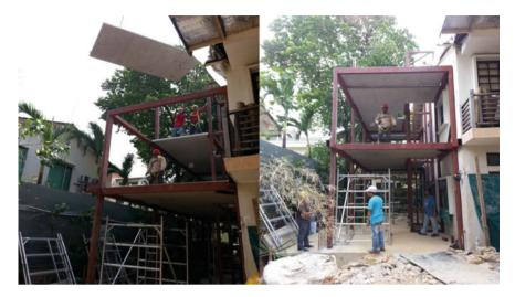
Fig. 6 Lifting and placing of pre-cast slabs onto modules
