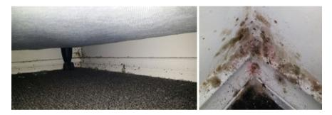
Fig. 20 Under the bed, the wall and carpet have limited exposure to the heating and experience thermal bridging to the external walls
