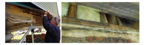
**Fig. 5** Often the true effect of condensation happens inside the wall framing. A builder helps dismantle the sheet metal cladding that is hard fixed against the studs (no battens) causing the wrap to be thermally bridged with the cold exterior. Indoor vapour, unable to pass through the foil wrap condenses on the insulation which acts as a reservoir, keeping the studs and bottom plate a moist breeding ground for mould
