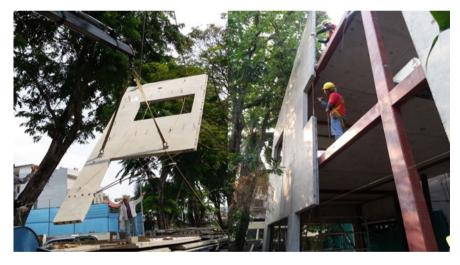
Fig. 7 Lifting of pre-cast wall and installing and clad onto modules at side elevation
